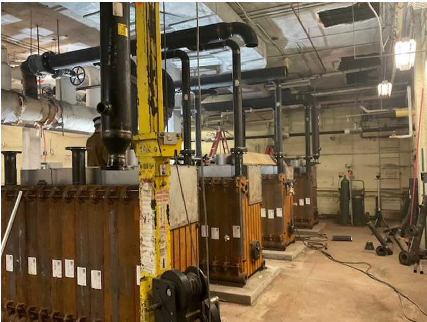
Boiler Room piping & valving installation continues. Estimated @ 50% Complete.
