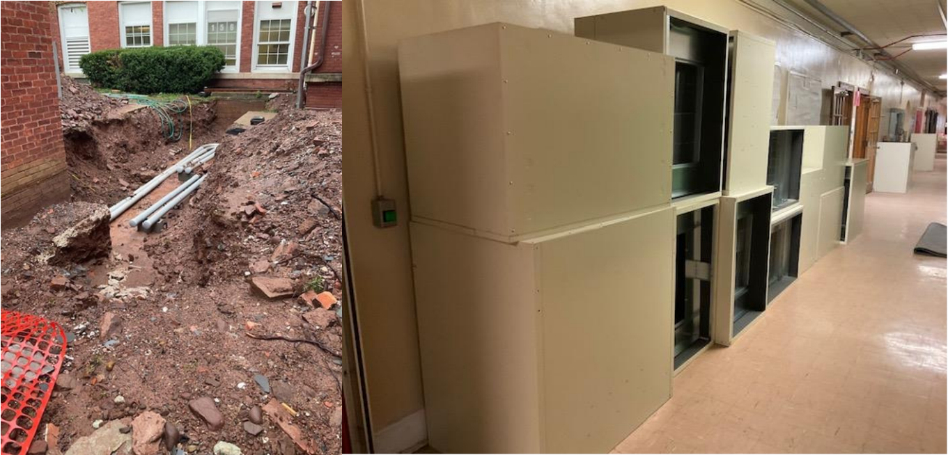
Left: Electric conduits for back feed of existing loads; Right: VUV Plenums
