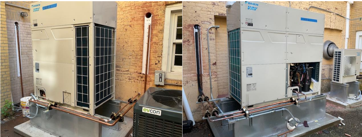
Courtyard Heat Pumps: Piping & wiring underway (not all shown). Refrigerant lines are being tested too.
