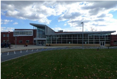
Exterior of building
