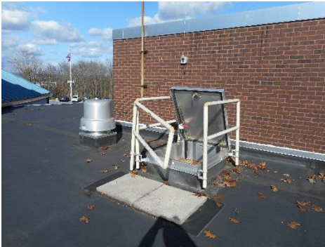
Gate at roof hatch
