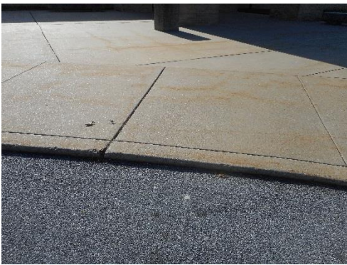
Curb at building entry
