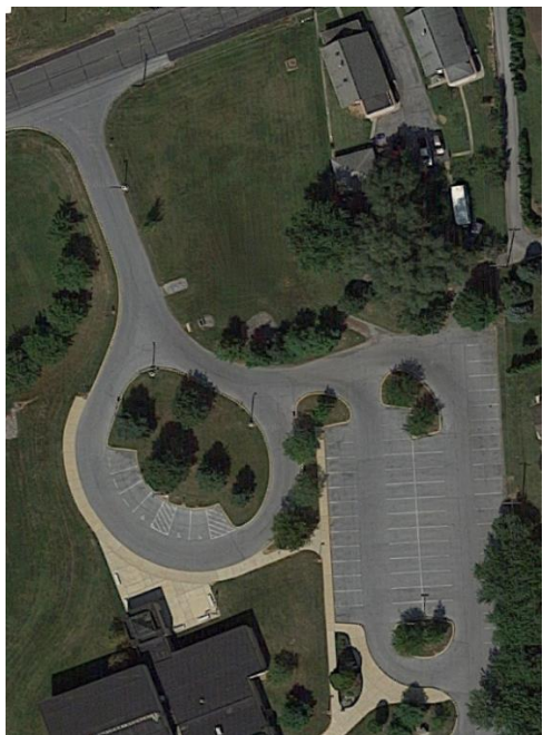
Flooding at parking access
