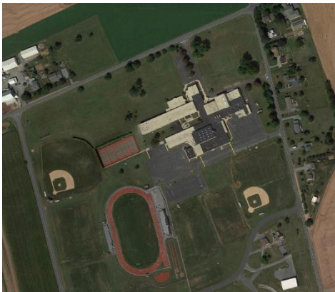
Aerial view of site
