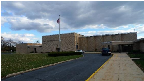
Bus loop at main entrance
