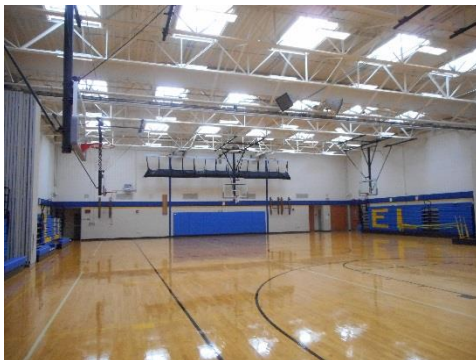
Gymnasium with natural light
