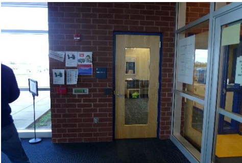
Secure entrance at vestibule
