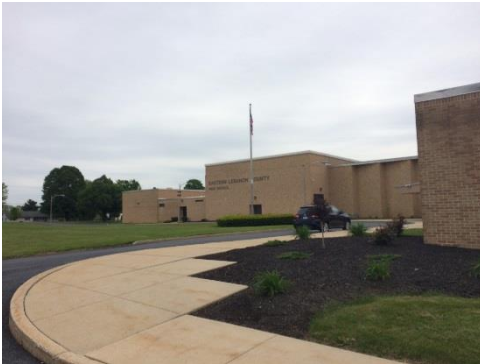
Exterior of building
