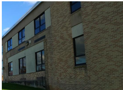
Typical exterior conditions
