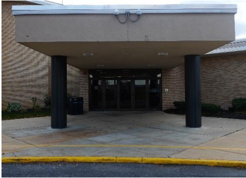
Main entrance to high school
