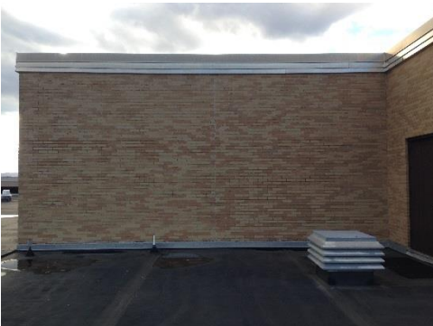
Typical flashing height at roof
