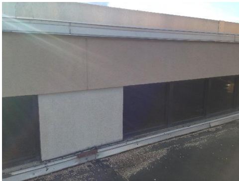
Roof at clerestory windows
