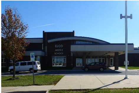
Exterior of building
