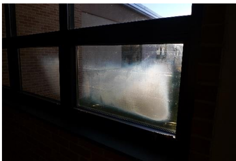
Seal failure on exterior glazing
