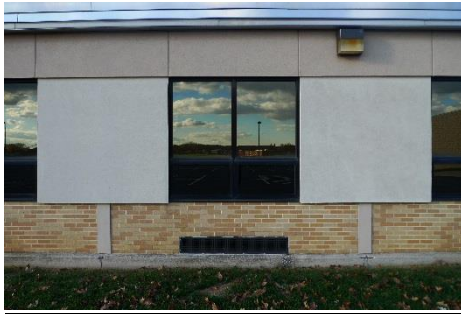
Typical exterior conditions
