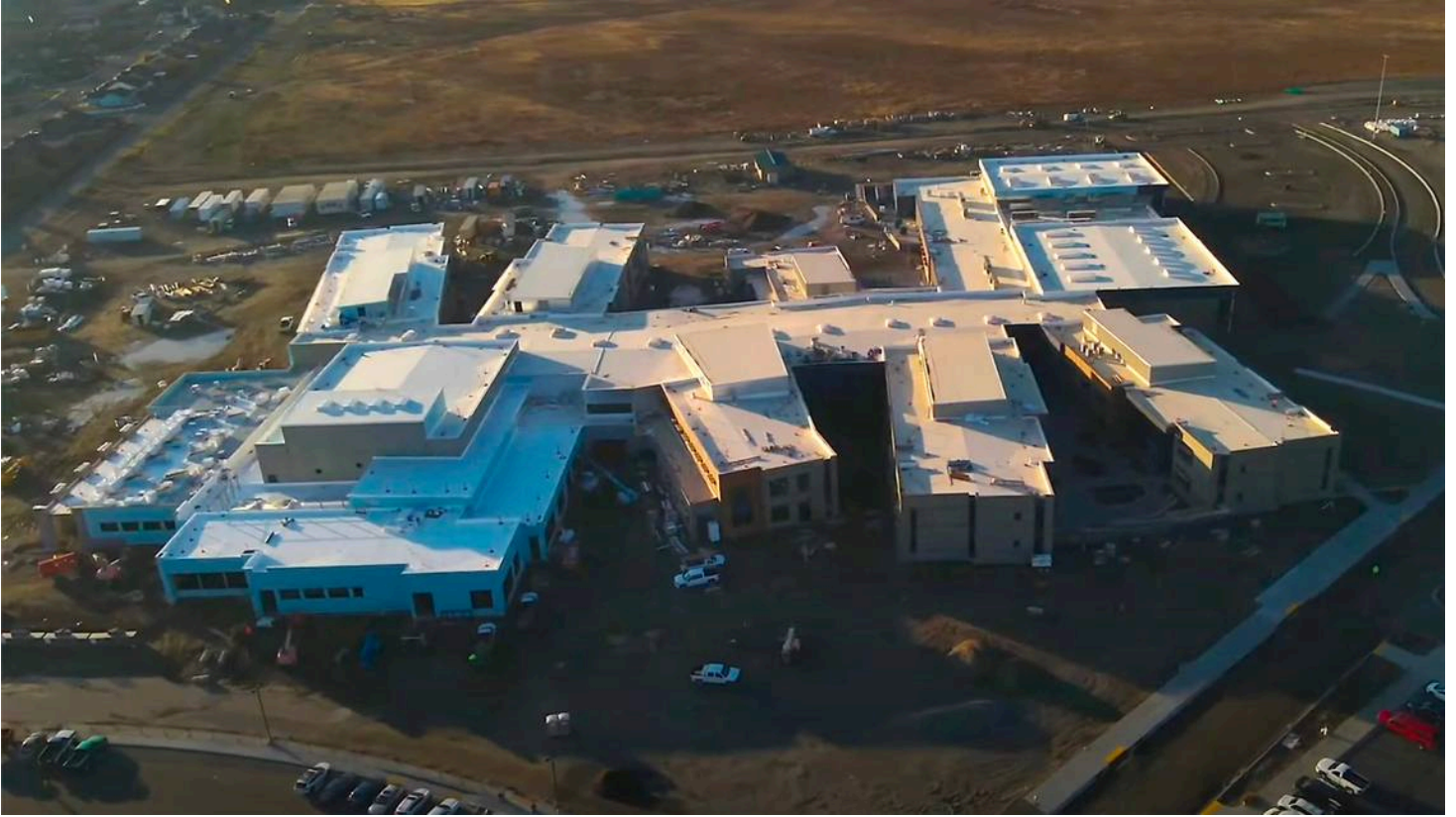
The $125 million school is set to open fall 2025 and will serve 2,000 students in west Pasco. Courtesy Pasco School District
