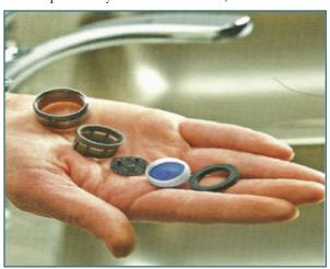
Rinse the pieces with water and brush off the debris. For deposits that are difficult to remove, soak the parts in water for a few minutes and scrub with a new toothbrush.
