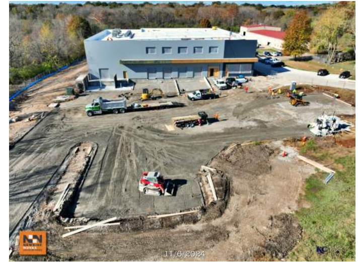
East Lot Construction
