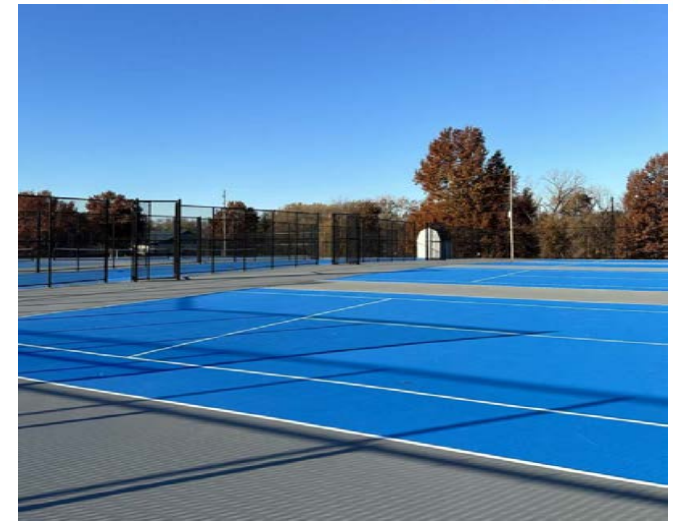
North Courts Looking Southwest
