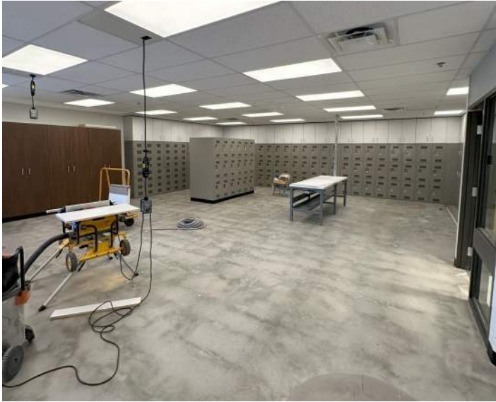
Progress 100's Wing
