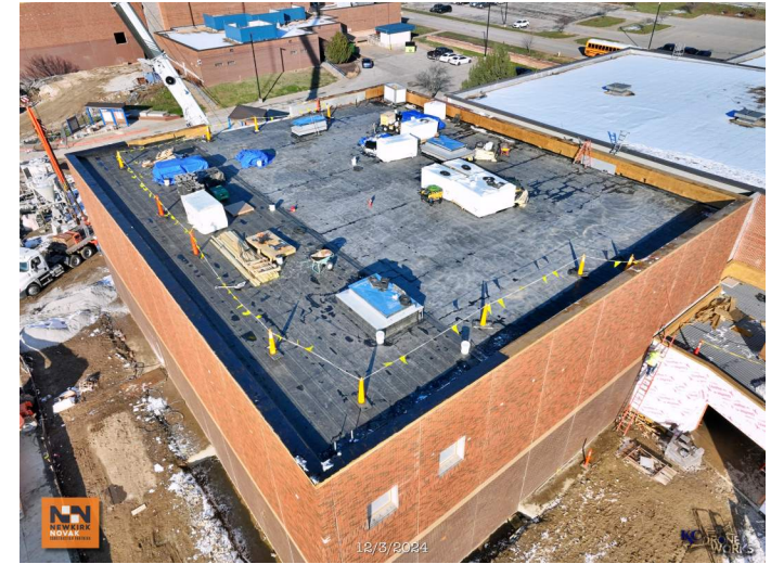
SVMS - Gym Roofing
