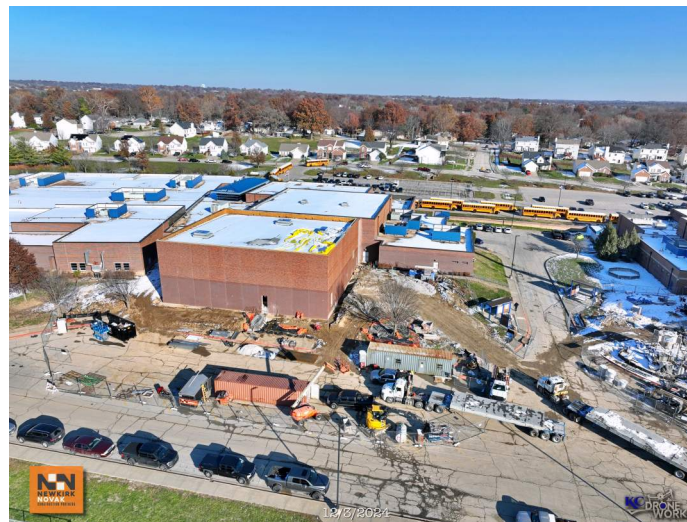
DMS - Pre-cast leave out panels installed
