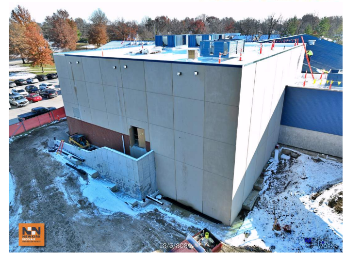
EPiC Elementary - N. Retaining Wall
