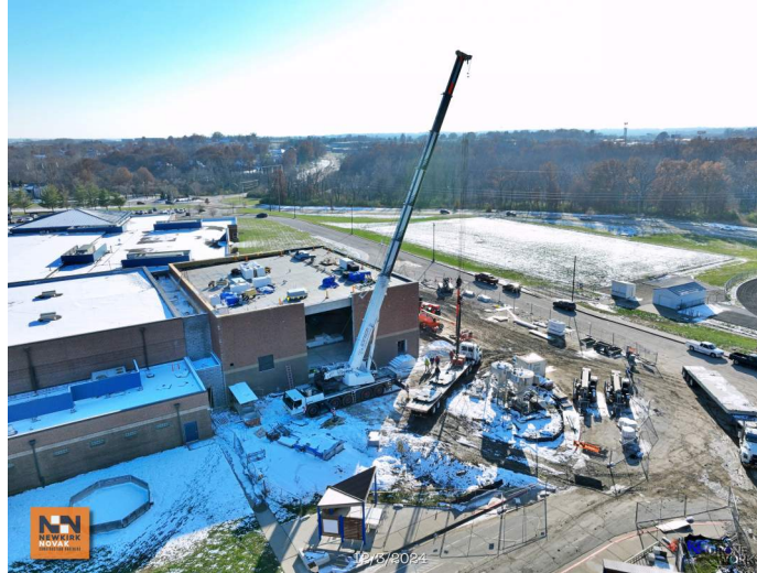
SVMS - Pre-cast panel leave out install
