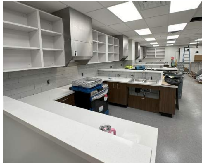
Progress 100's Wing
