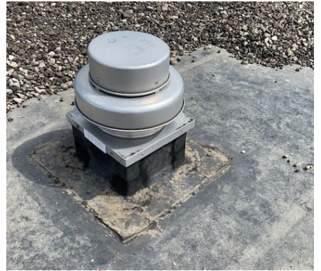
Flashing for rooftop equipment failing due to shrinking roof materials.
