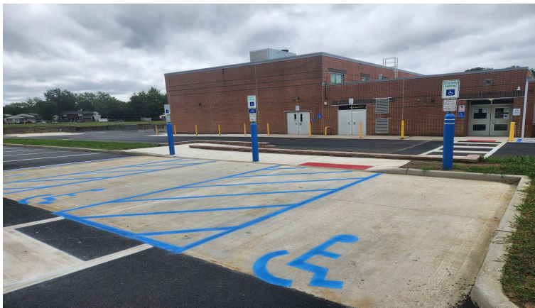
Sitework at Woodcrest
