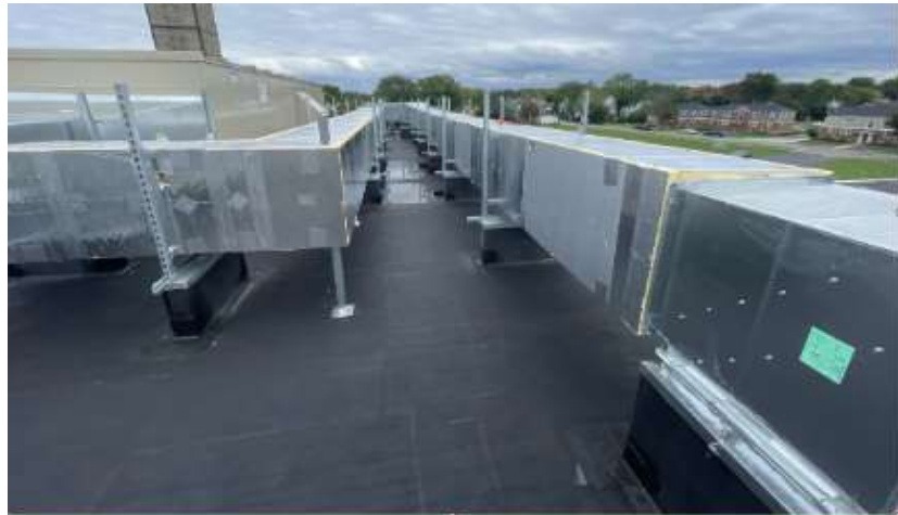
WBS - New Auditorium RTU + assoc. ductwork
