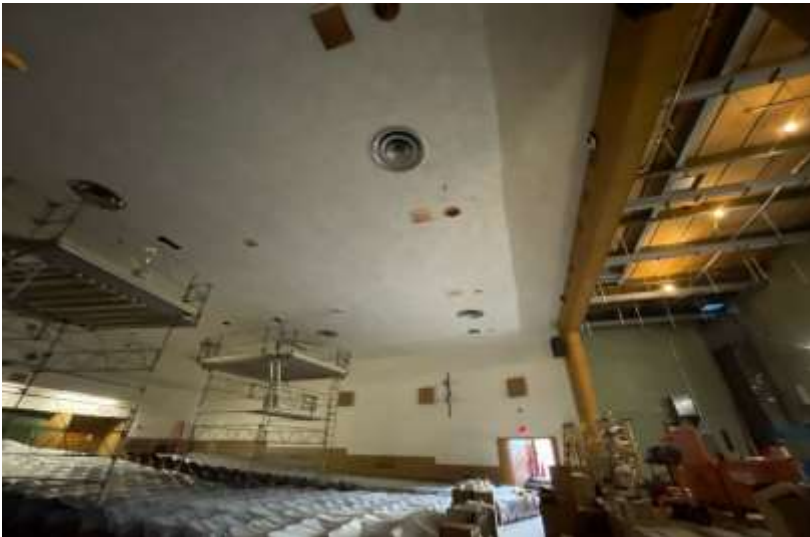
WBS - Aud. structural steel for new theatrical rigging & high-volume-low-speed fans
