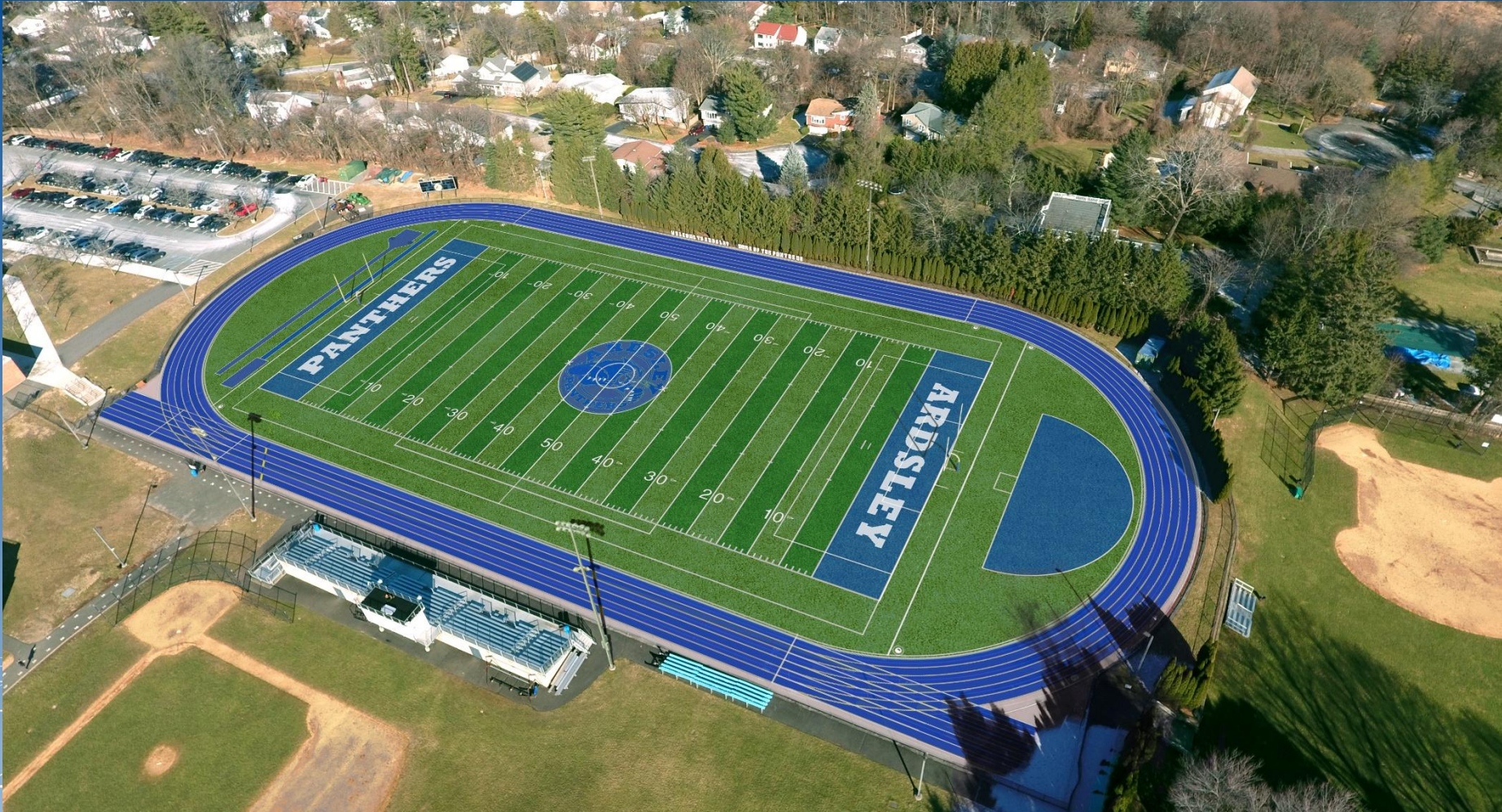
PROJECT #1 - High School Track, Synthetic Field and Lights
