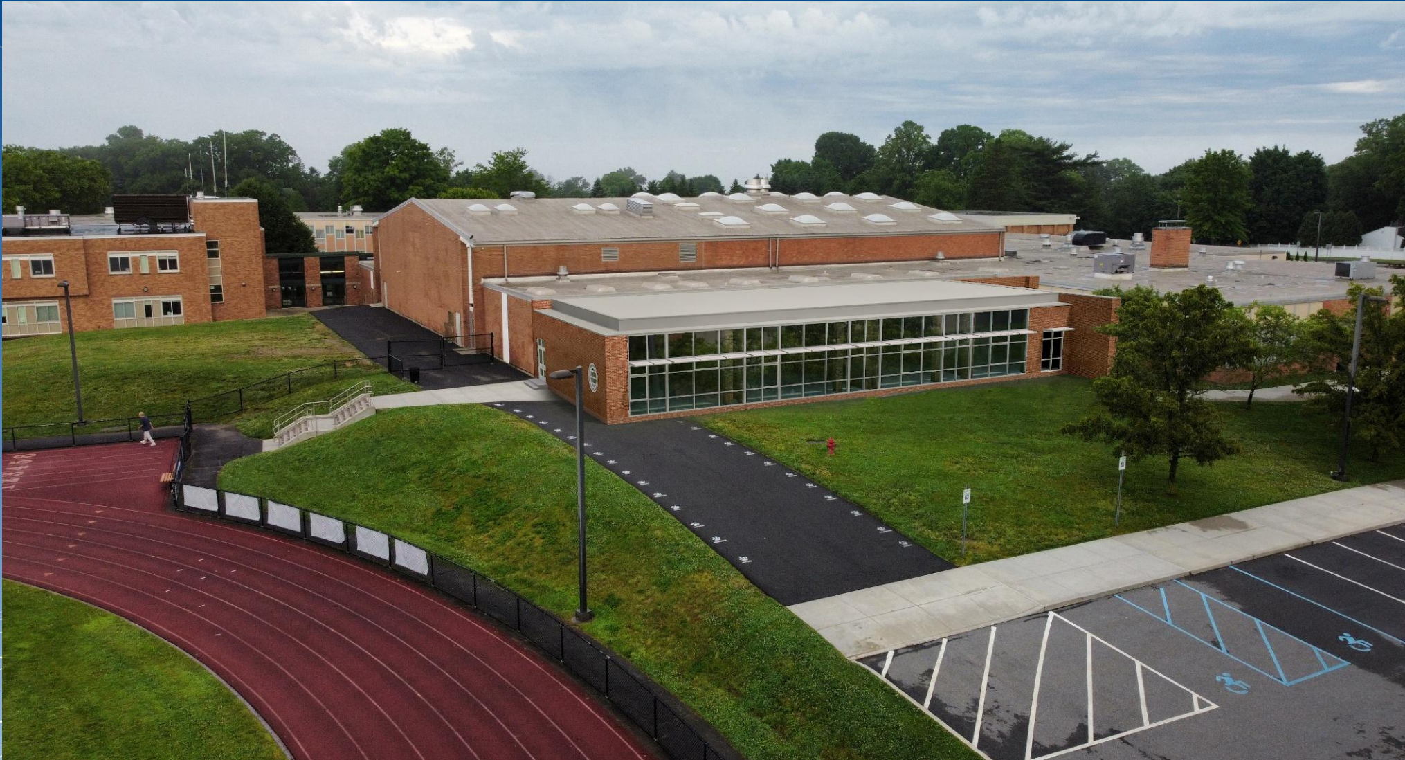
PROJECT #2 - High School New Four Classrooms Addition with Renovated Restrooms
