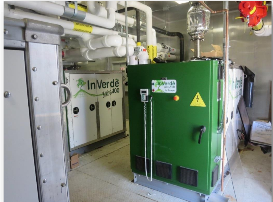
Johnson Controls Installation of 100 kW Cogeneration Unit at Eastport School District
