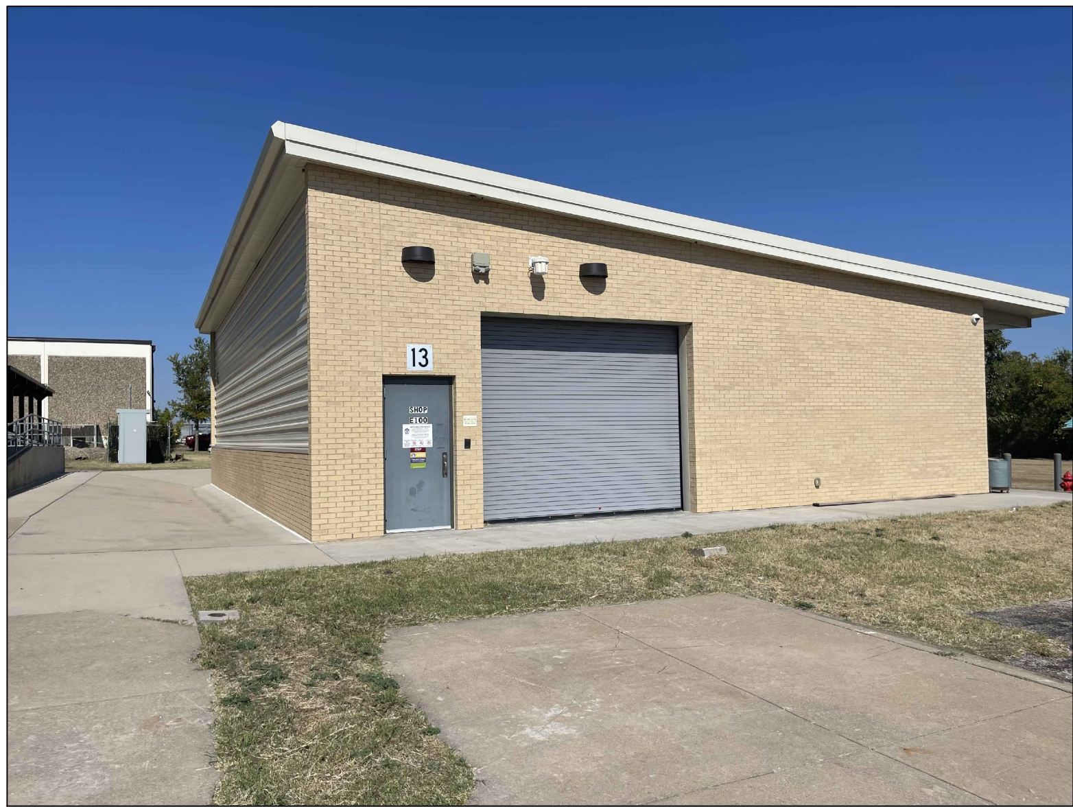
PICTURE: EXISTING SHOP BUILDING EXTERIOR
