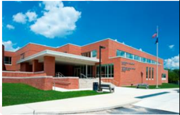
Slatington Elementary School (3-6)
