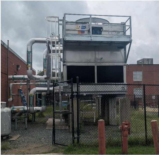
Brooke Point High School: Cooling Tower Replacement
