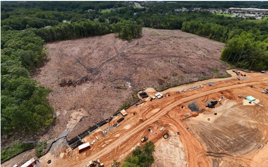
Elementary #18: Site Clearing
