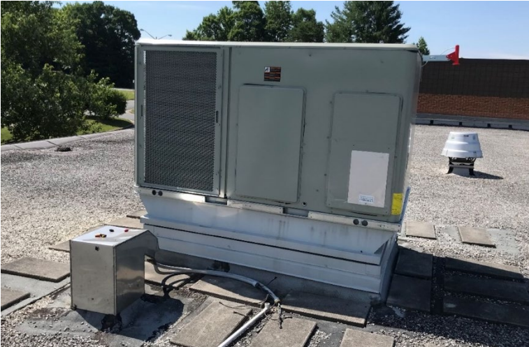
Park Ridge Elementary: Mechanical Equipment Replacement
