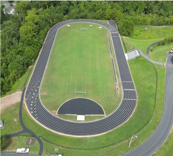
Dixon-Smith Middle: Track Repair
