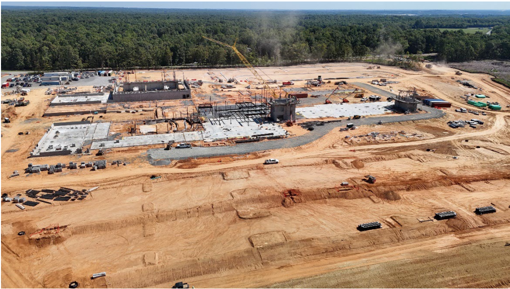
High School #6: Under Construction
