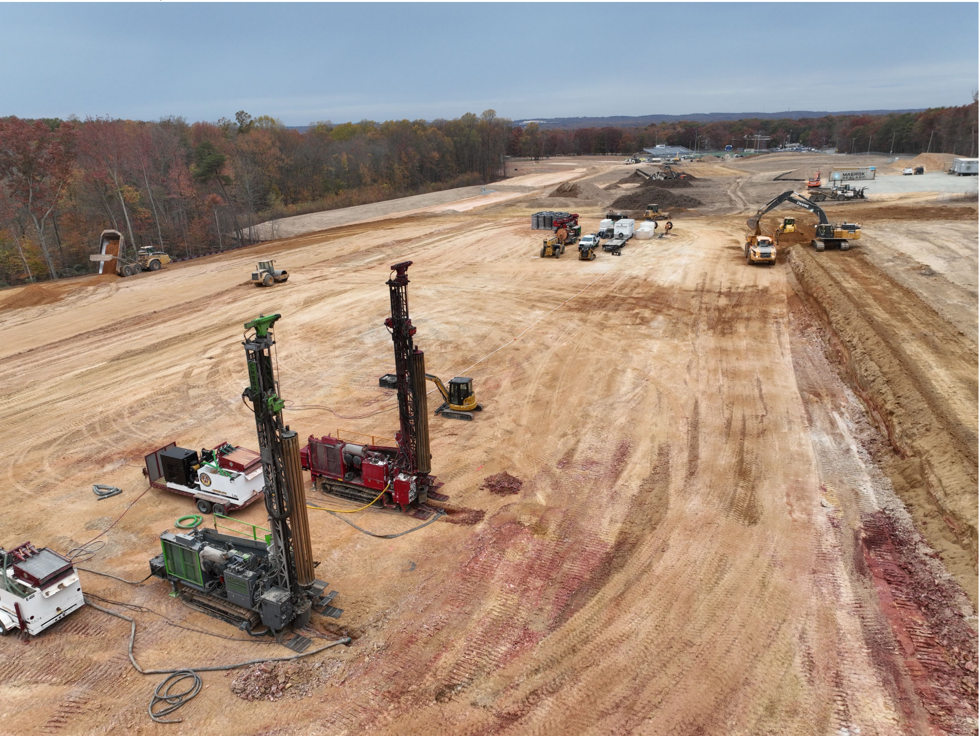
NORTH EAST MIDDLE / HIGH SCHOOL – GEOTHERMAL WELLS DRILLING
