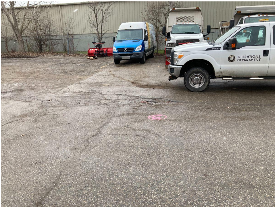
Photograph No. 4: High severity block, fatigue, transverse and longitudinal cracking near boring B-6. View to the south.
