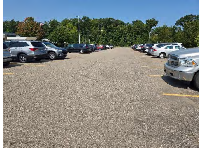
Photograph No. 14: Low severity block and fatigue cracking looking north from B-4
