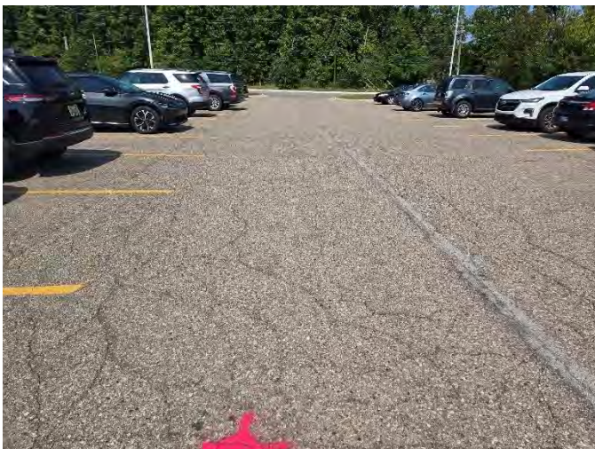
Photograph No. 17: Low to moderate severity fatigue and longitudinal cracking looking north from B-5
