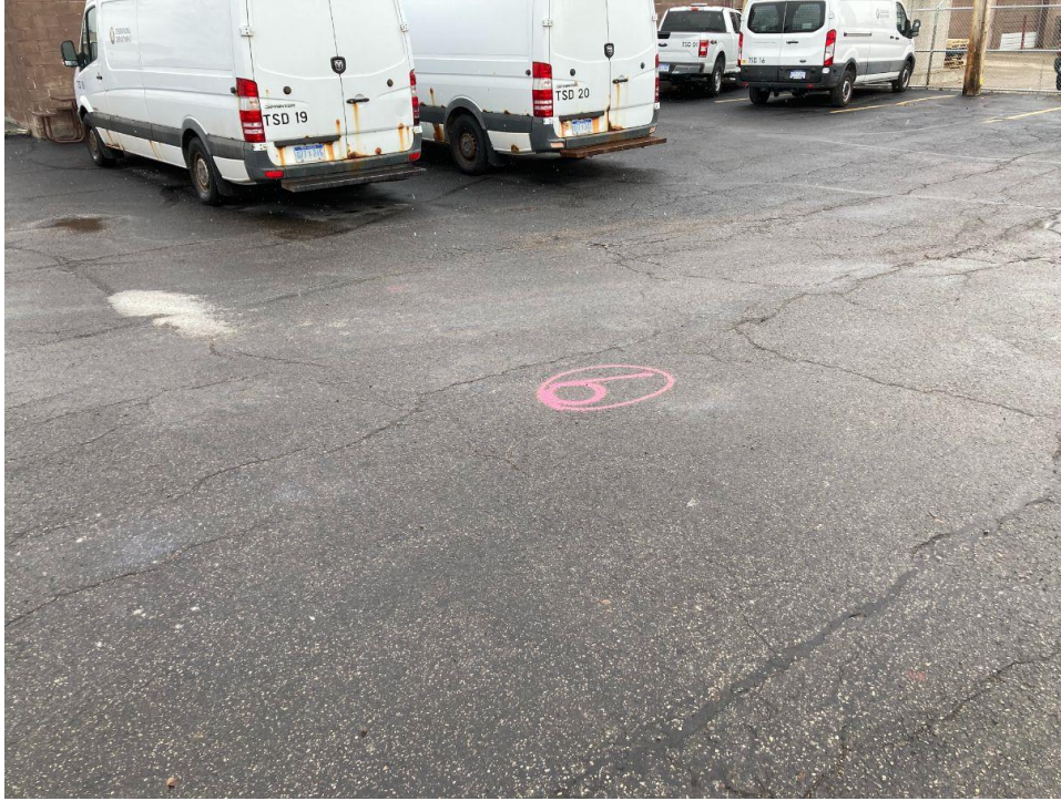
Photograph No. 7: Moderate to high severity transverse, longitudinal, and fatigue cracking near boring B-9. Crack sealing in one area. View to the northeast.
