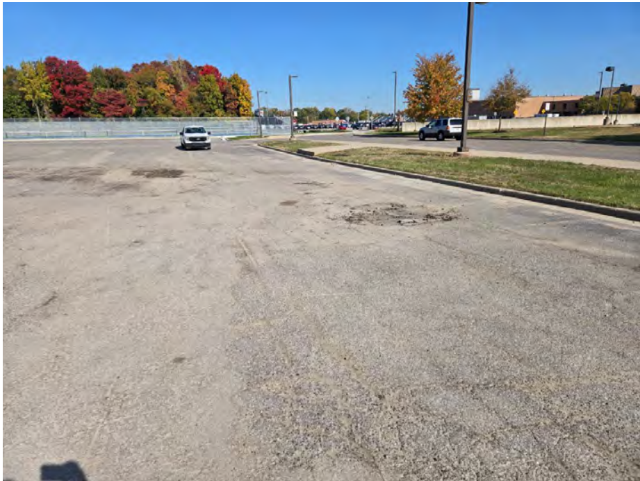
Photograph No. 22: Potholes and pavement raveling along east lot, looking north
