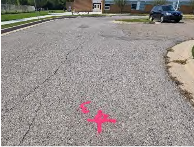
Photograph No. 13: Moderate severity fatigue cracking near B-3
