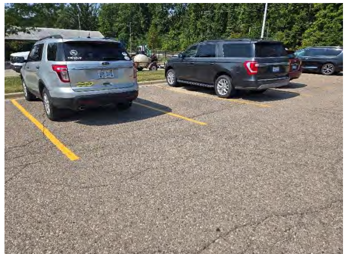
Photograph No. 18: Low to moderate severity fatigue cracking behind parking stalls
