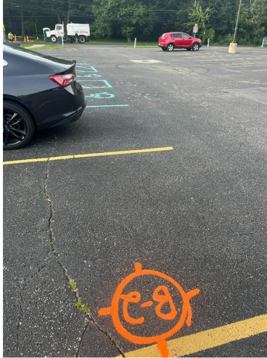
Photograph No. 3: Looking south, low to moderate severity block and fatigue cracking.
