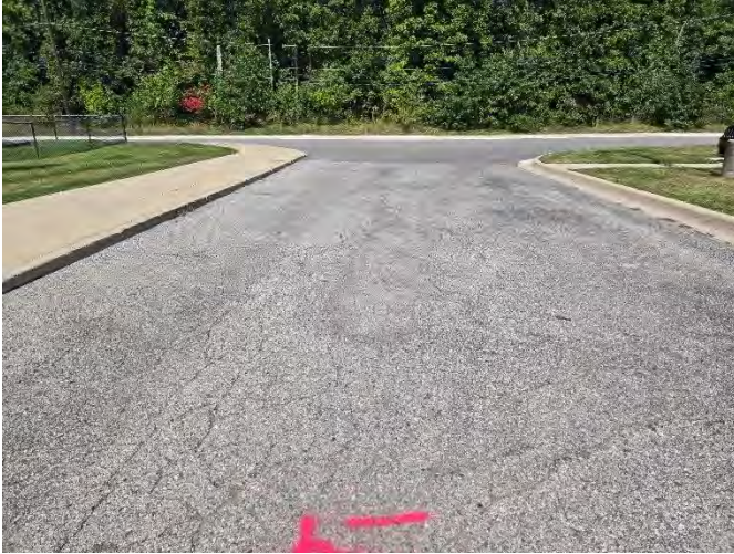
Photograph No. 1: Moderate severity fatigue cracking, looking north from B-1
