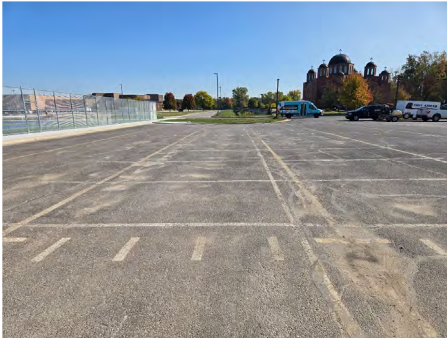
Photograph No. 17: Looking east toward B-65, moderate severity block and fatigue cracking and sediment indicating settlement of subgrade and previous ponding
