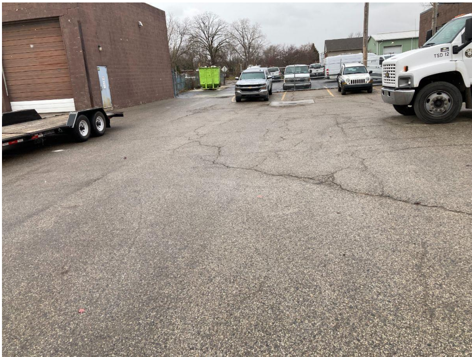
Photograph No. 6: Moderate severity transverse and longitudinal cracking near boring B-8. View to the west.
