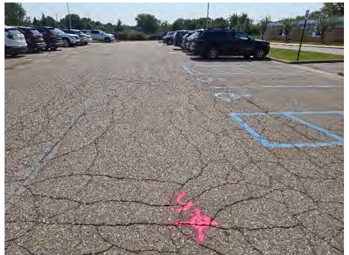
Photograph No. 16: Moderate severity fatigue cracking looking south at B-5
