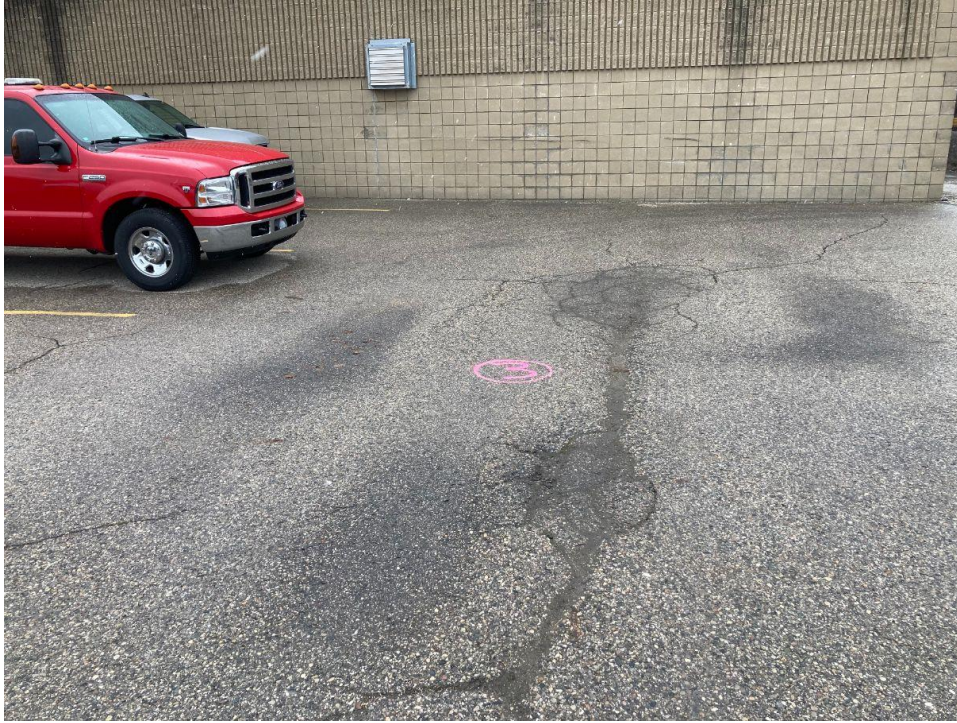
Photograph No. 1: Moderate severity fatigue cracking and evidence of settlement near boring B-3. View to the south.
