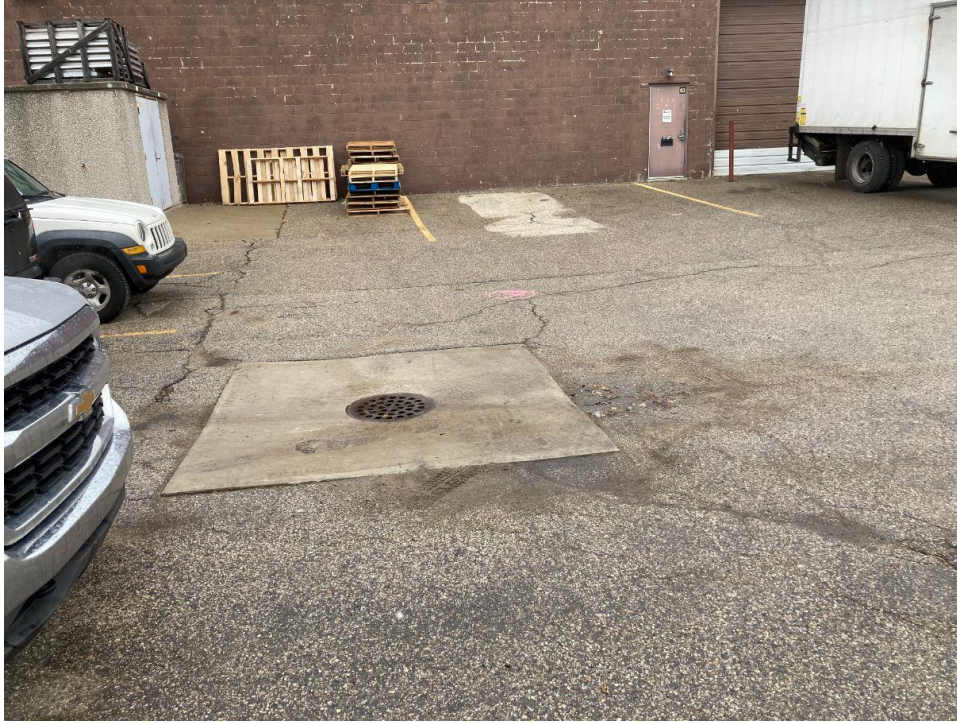
Photograph No. 5: Low to moderate severity transverse and longitudinal cracking near boring B-7. Concrete collar around basin. View to the north.
