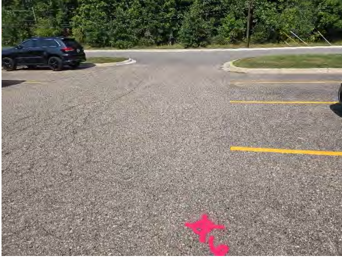
Photograph No. 19: Moderate severity fatigue cracking in center lot looking north at B-6
