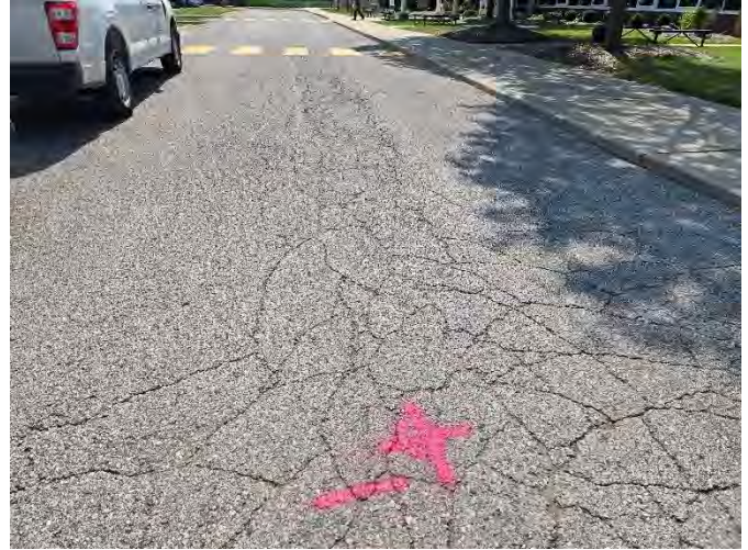
Photograph No. 2: Moderate severity fatigue cracking, looking south at B-1
