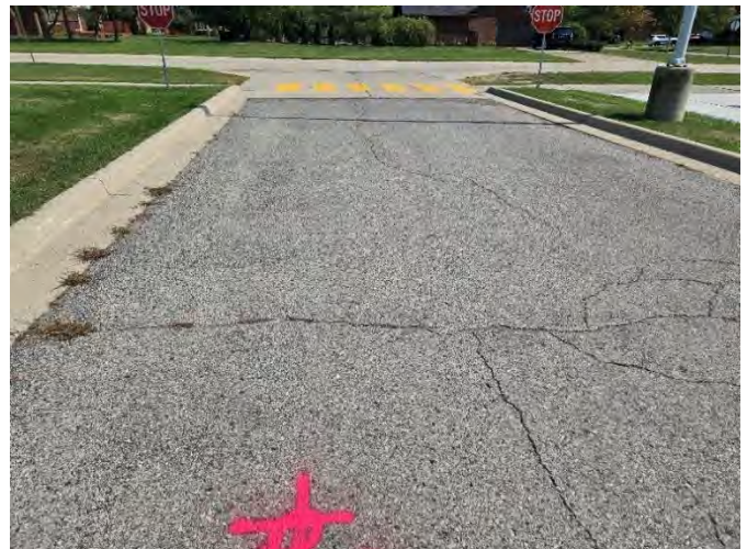
Photograph No. 12: Low severity transverse and fatigue cracking at south entrance.
