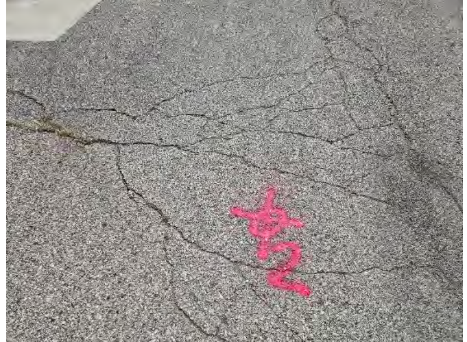
Photograph No. 8: Low severity fatigue cracking near B-2
