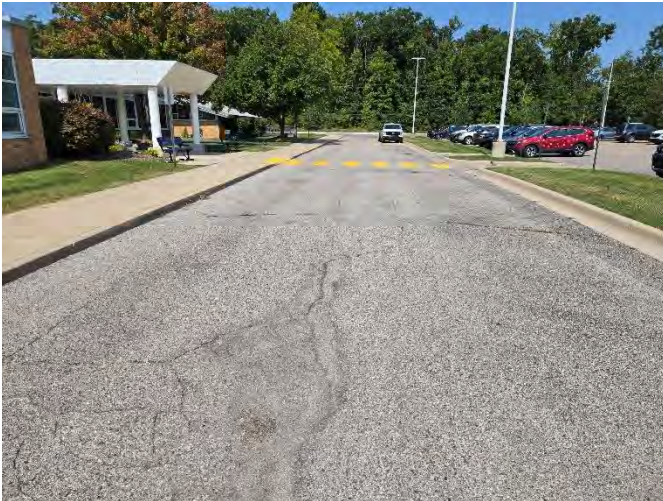
Photograph No. 9: Low severity block and fatigue cracking north of B-2
