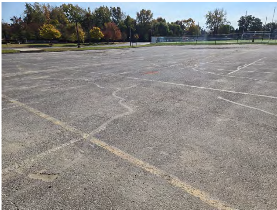
Photograph No. 18: Looking southeast toward B-66, moderate severity block and fatigue cracking, pavement surface raveling
