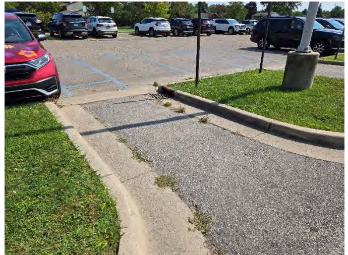
Photograph No. 4: Drainage structure in gutter
