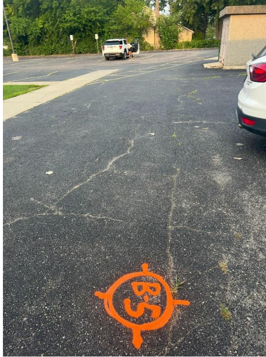
Photograph No. 9: Low to moderate severity fatigue cracking looking west.
