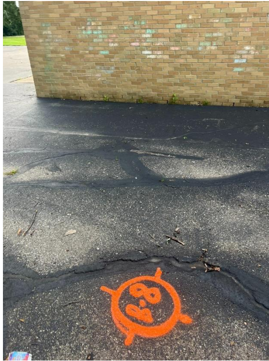
Photograph No. 15: Pavement flush to building. Moderate to high severity cracking.
