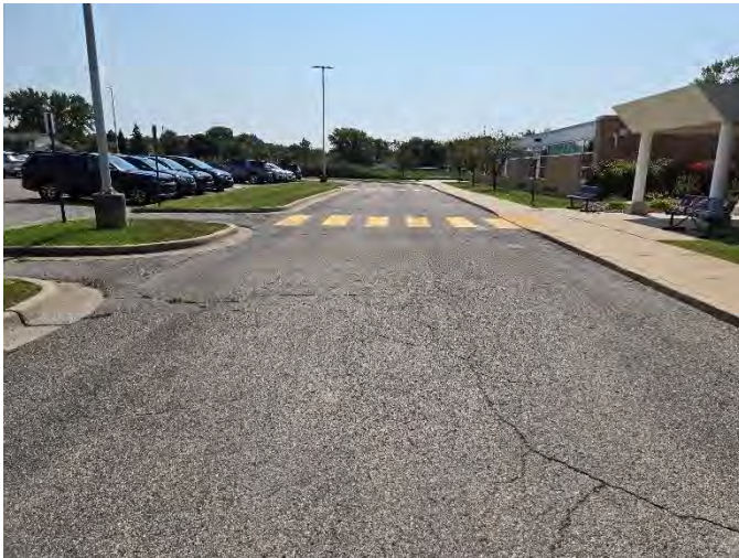
Photograph No. 3: Low severity block and fatigue cracking, south of B-1
