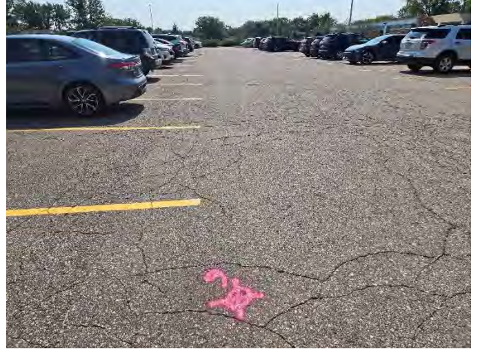
Photograph No. 20: Moderate severity fatigue cracking in center lot looking south at B-6
