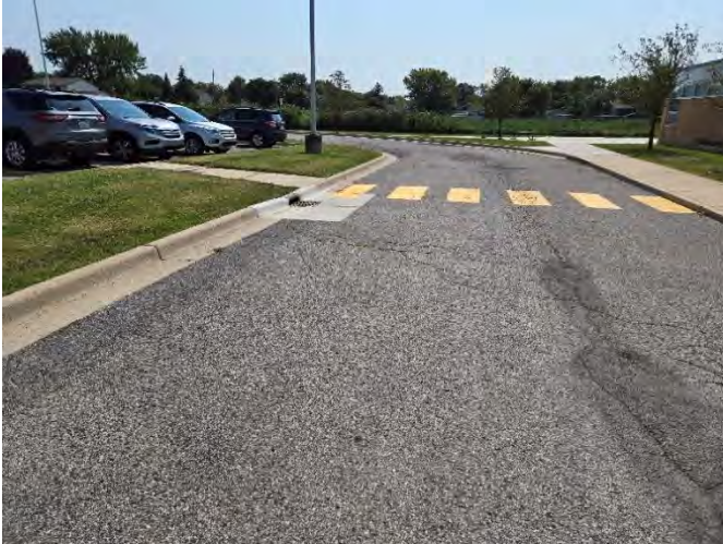
Photograph No. 7: Low to moderate severity block cracking near B-2. New concrete around drainage structure.
