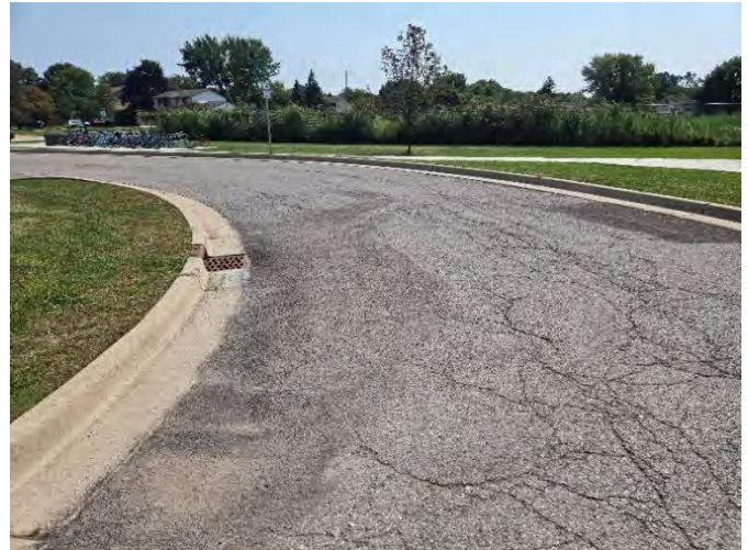
Photograph No. 10: Moderate severity fatigue cracking south of B-2. Sediment along gutter.
