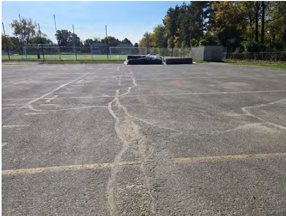
Photograph No. 19: Looking south toward B-67, moderate severity block and fatigue cracking and pavement raveling
