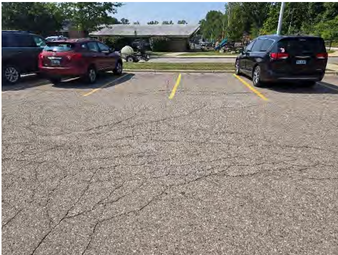
Photograph No. 21: Moderate severity fatigue cracking in center lot looking south at B-6
