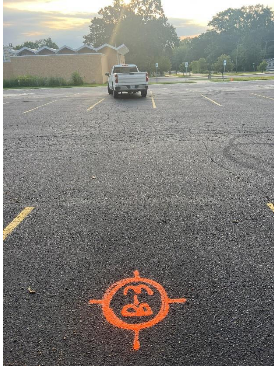
Photograph No. 5: Moderate to high severity fatigue cracking through center of drive lane, looking east.
