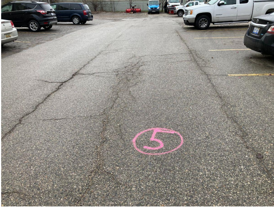
Photograph No. 3: Moderate severity transverse, longitudinal, and fatigue cracking near boring B-5. View to the south.
