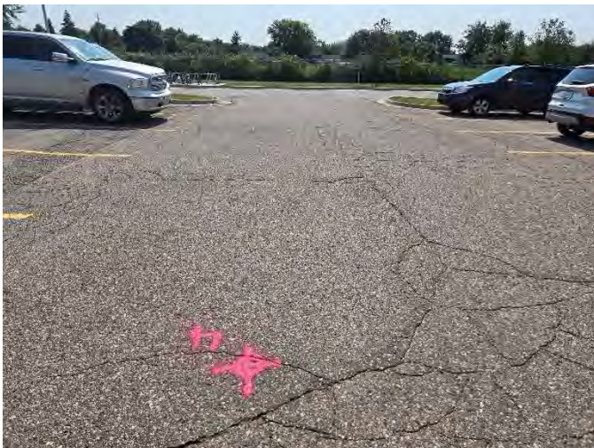
Photograph No. 15: Moderate severity fatigue cracking looking south at B-4
