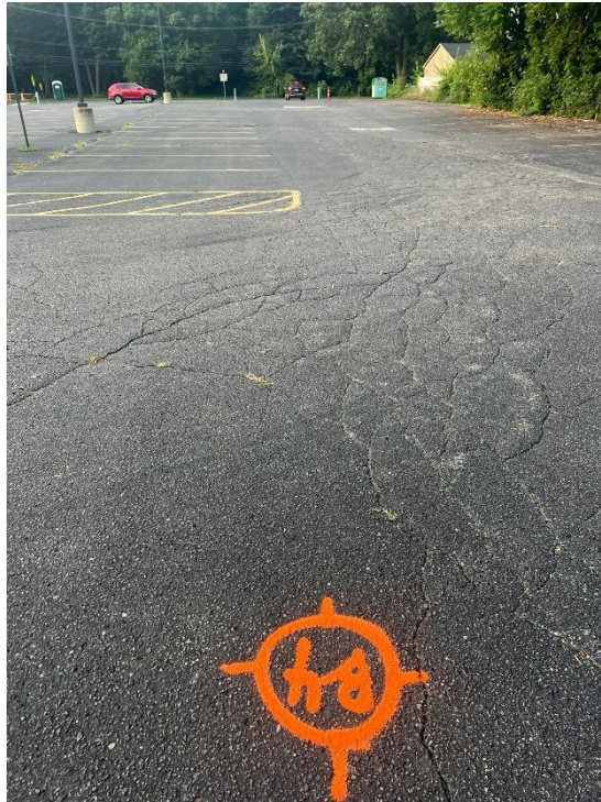
Photograph No. 8: Moderate to high severity fatigue cracking looking south.
