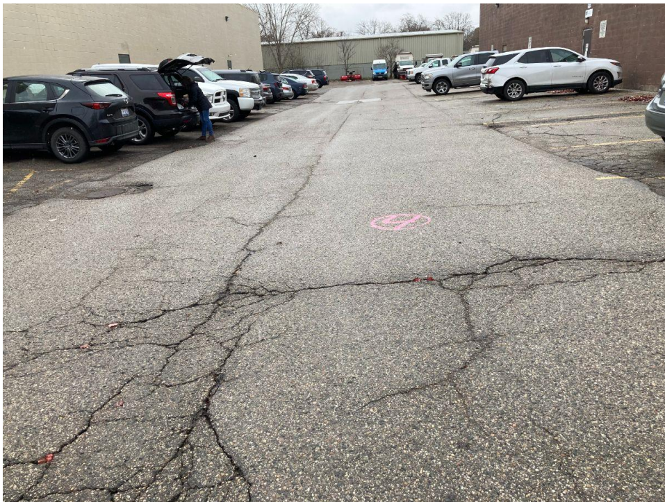
Photograph No. 2: Moderate to high severity transverse, longitudinal, and fatigue cracking near boring B-4. View to the south.
