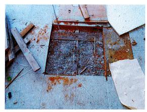
3. Steel bar joist, with what appears to be gypsum panels, was observed in the north end of the building.
