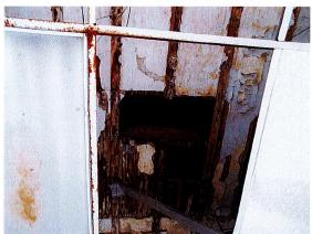
4. Water has infiltrated the building in the north east corner. Wood roof framing is damaged.
