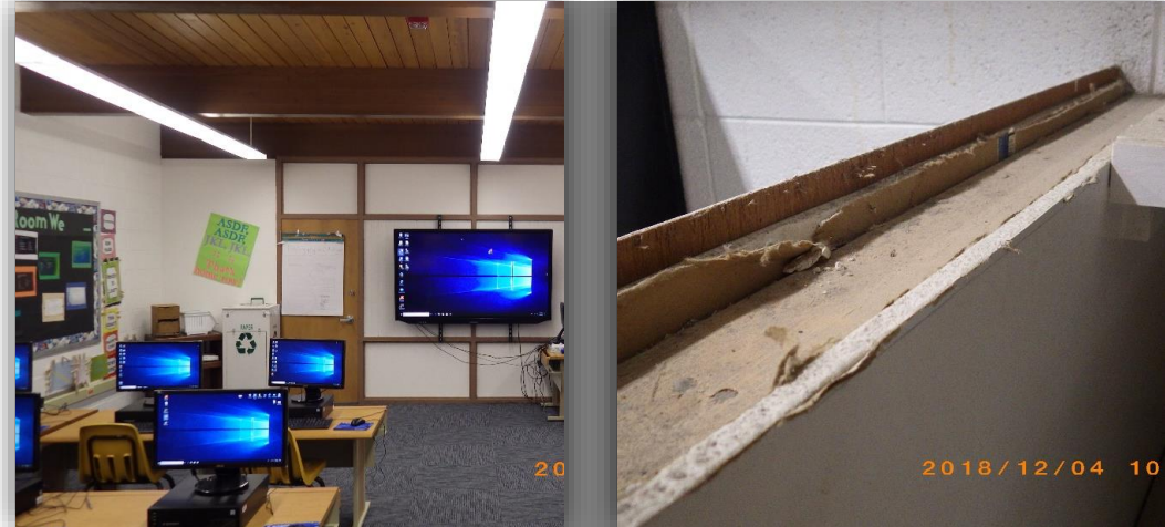
No Fire Suppression System Wood Framed Walls Not Allowed
