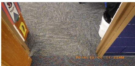
Square tile in classroom abutting broadloom carpet (roll) carpet at the corridor
