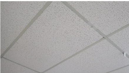
2x4 ATC ceiling tile and grid at classroom.
