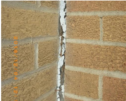
Deteriorated joint sealant
