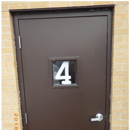
Hollow metal frame & door; peeling paint on lintel
