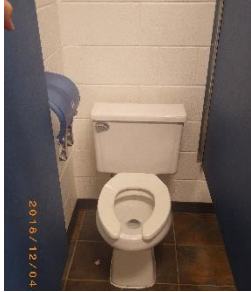
Stall is not ADA compliant
