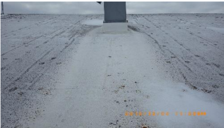
Plastic singly-ply roof membrane over gym
