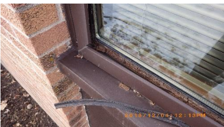
Rotted sash at exterior window
