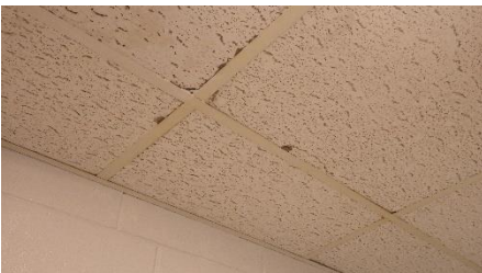
Discolored 2x4 ATC ceiling tile and grid
