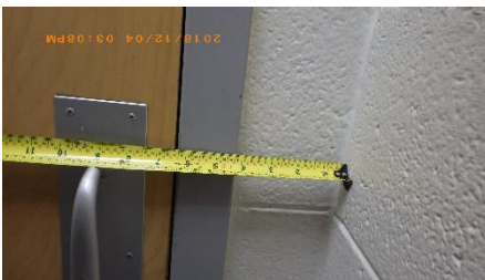
Clear area / pull space at door less than 12"
