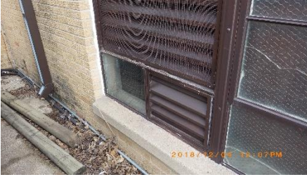
Original steel frame window with broken glazing
