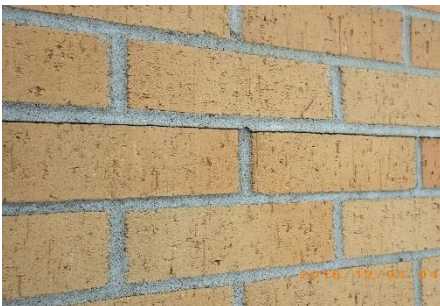
Example of mortar joint with hairline crack
