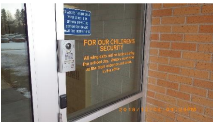
Signage & video-intercom at main entry
