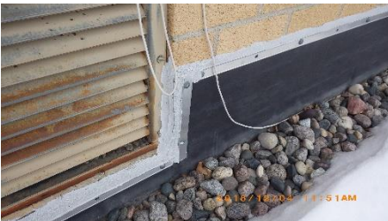
Rust at louver, deteriorating sealant at roof
