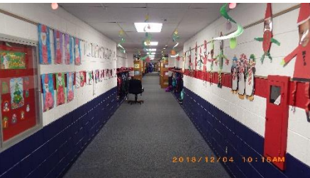
CMU walls and 2x4 ATC ceiling at 1954 corridor
