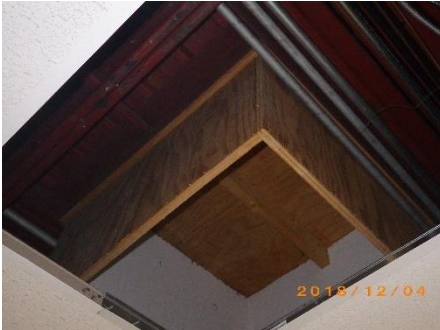
Steel roof deck / abandoned skylight
