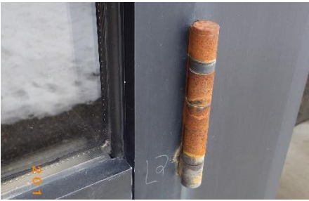
Rusted hinge at aluminum entrance door
