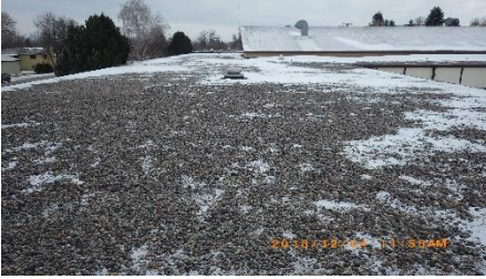
Ballasted EPDM roof
