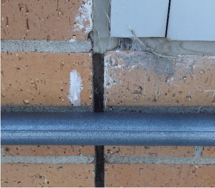
Aluminum window with missing sealant under vertical framing; control joint below window with no mortar or sealant
