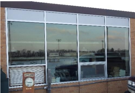
Aluminum window with insulated glazing
