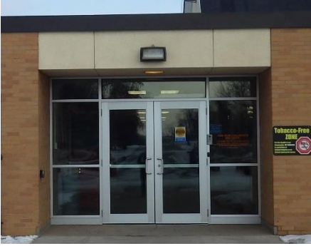
Aluminum entrance door with plaster soffit
