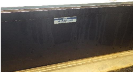
Condensation on interior side of aluminum
