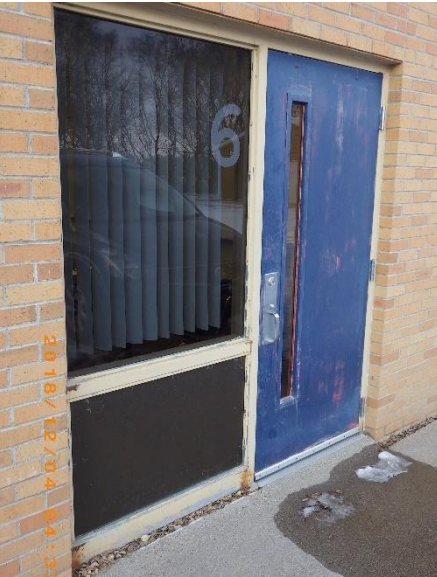
Hollow metal frame/door with rust and faded paint
