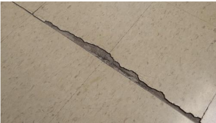
Deteriorated VCT flooring at main corridor
