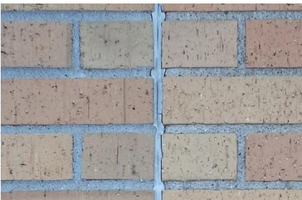
Deteriorated sealant at masonry control joint
