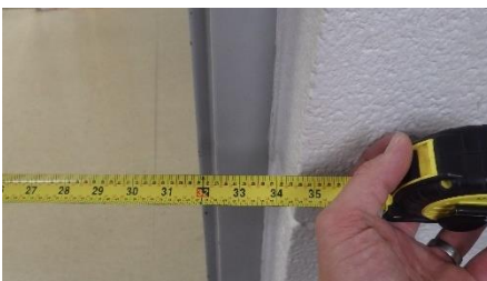
Door widths less than 36" wide
