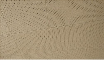
Perforated acoustical metal tile at kitchen
