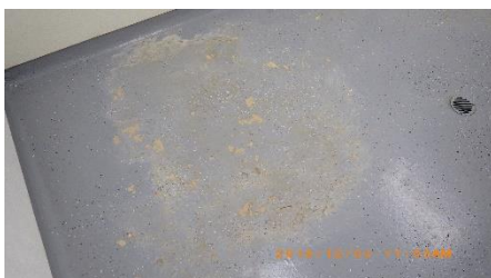
Painted floor at shower is deteriorated, peeling.
