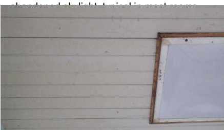
Tongue and groove (T&G) ceiling with
