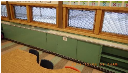
Original casework at exterior wall that is part of the cabinet unit ventilator (CUV)
