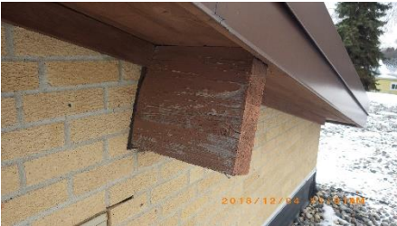
Peeling paint at wood beams and deck
