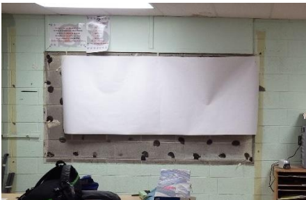
Glue pucks on wall may have asbestos
