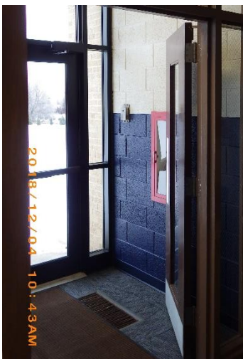
Vestibule doors do have proper floor clearance and not ADA compliant
