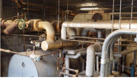
Pipe elbows, boiler insulation with asbestos
