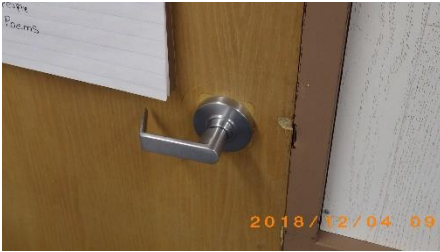
ADA compliant lever style door hardware
