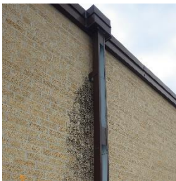
Downspout at roof edge with staining on brick
