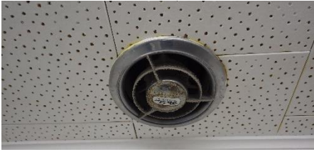
12x12 acoustical tile (may have asbestos glue)
