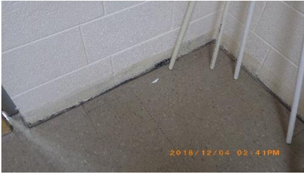
Vinyl Asbestos Tile
