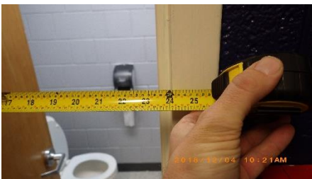
Door opening is not ADA compliant
