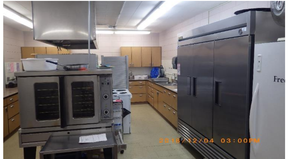
Vinyl Asbestos Tile
