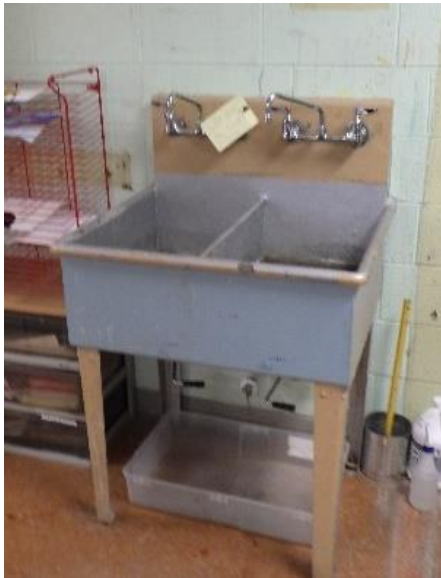
Shop sink with no plumbing drain pipe.
