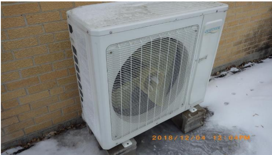
AC Unit Improperly Supported.
