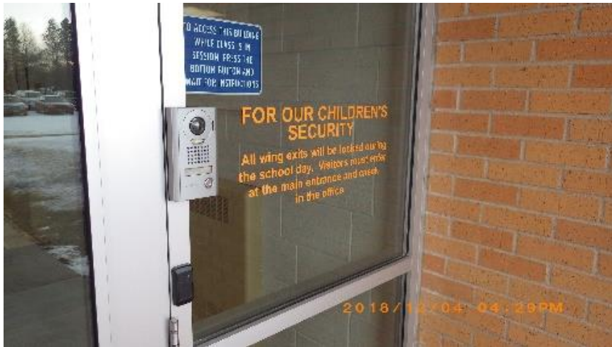
Signage & video-intercom at main entry
