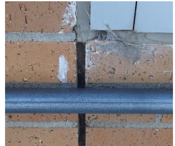
Missing Sealant
