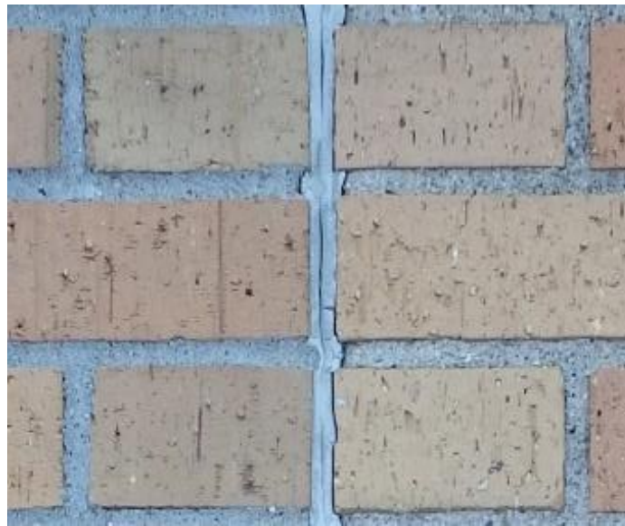
Deteriorated Sealant
