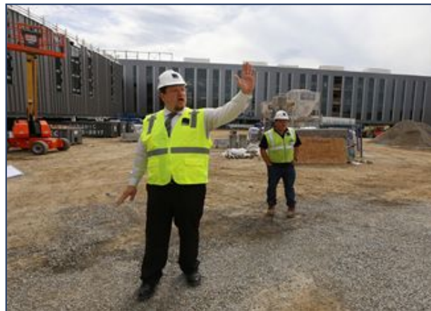
BILLERICA SUPERINTENDENT AND CHAIR OF VALLEY COLLABORATIVE'S BOARD OF DIRECTORS TIM PIWOWAR OVERSEES CONSTRUCTION AT THE NEW BILLERICA HIGH SCHOOL.
