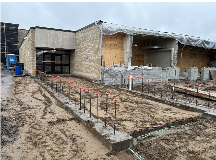
FINISH FOUNDATION WALLS FOR EAST ADDITION
