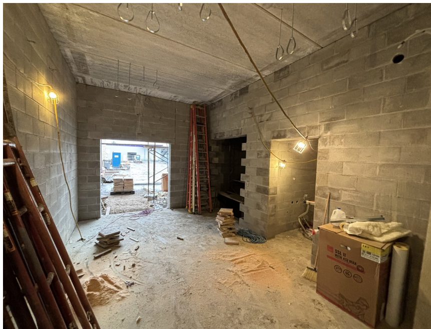
TEMP LIGHTING INSTALLED IN ELEVATOR
