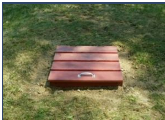
INSIDE AND OUTSIDE VIEWS OF THE ROOT CELLAR OUR TEAM BUILT AND INSTALLED UNDERGROUND. THE ROOT CELLAR INCLUDES A CUSTOM VALLEY COLLABORATIVE LOGO.
