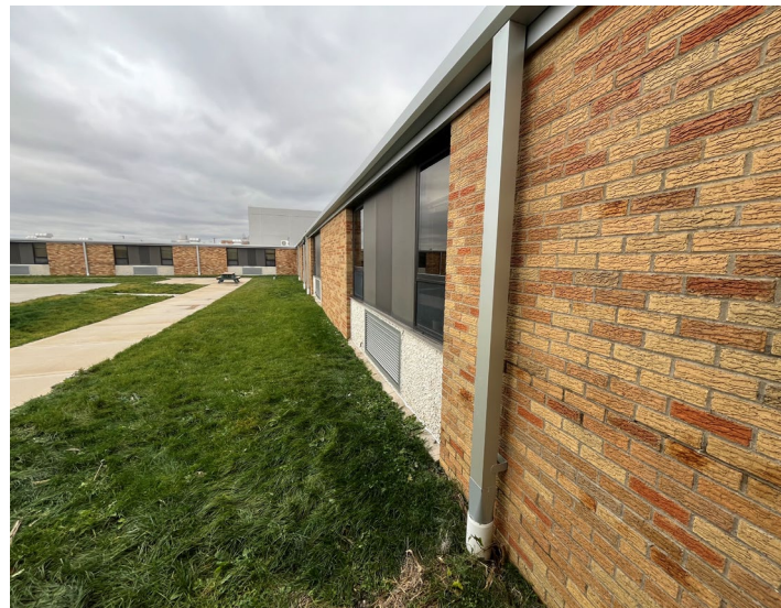
Gutter Installation
