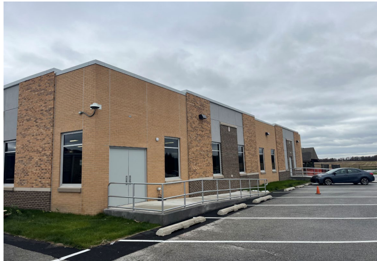
Metal Coping on New Cafeteria
