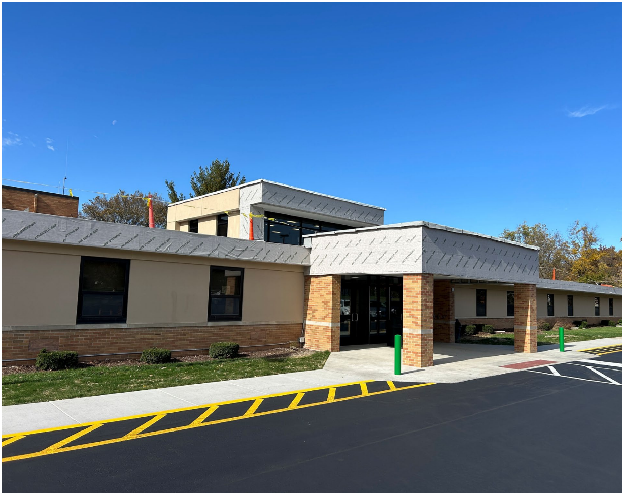
New Clerestory/Roofing Progress
