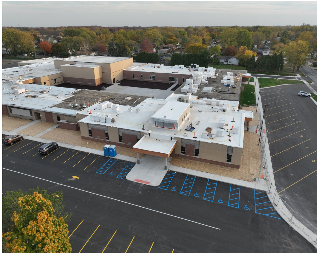
Unit A Progress
