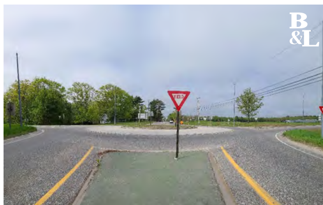
Figure 26 - Example of a Single Lane Roundabout Design
