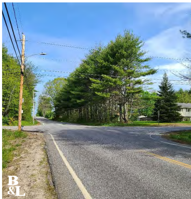
Figure 21 - Intersection of Broadturn Road at Burnham Road, Street View facing North
