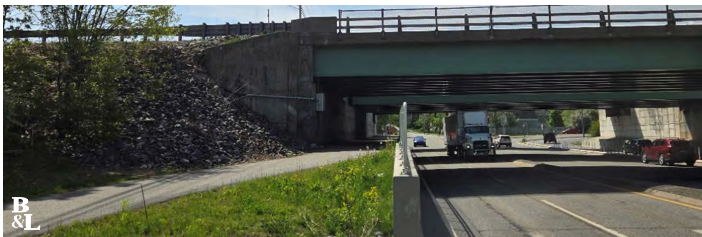
Figure 19 - Example of a Raised Pedestrian Walkway underneath an Overpass, Street View
