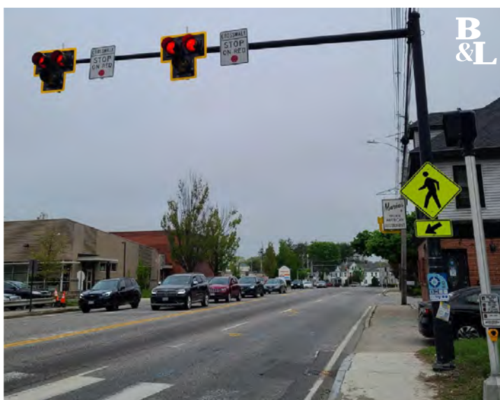
Figure 15 - Example of a Pedestrian Beacon/HAWK Signal
