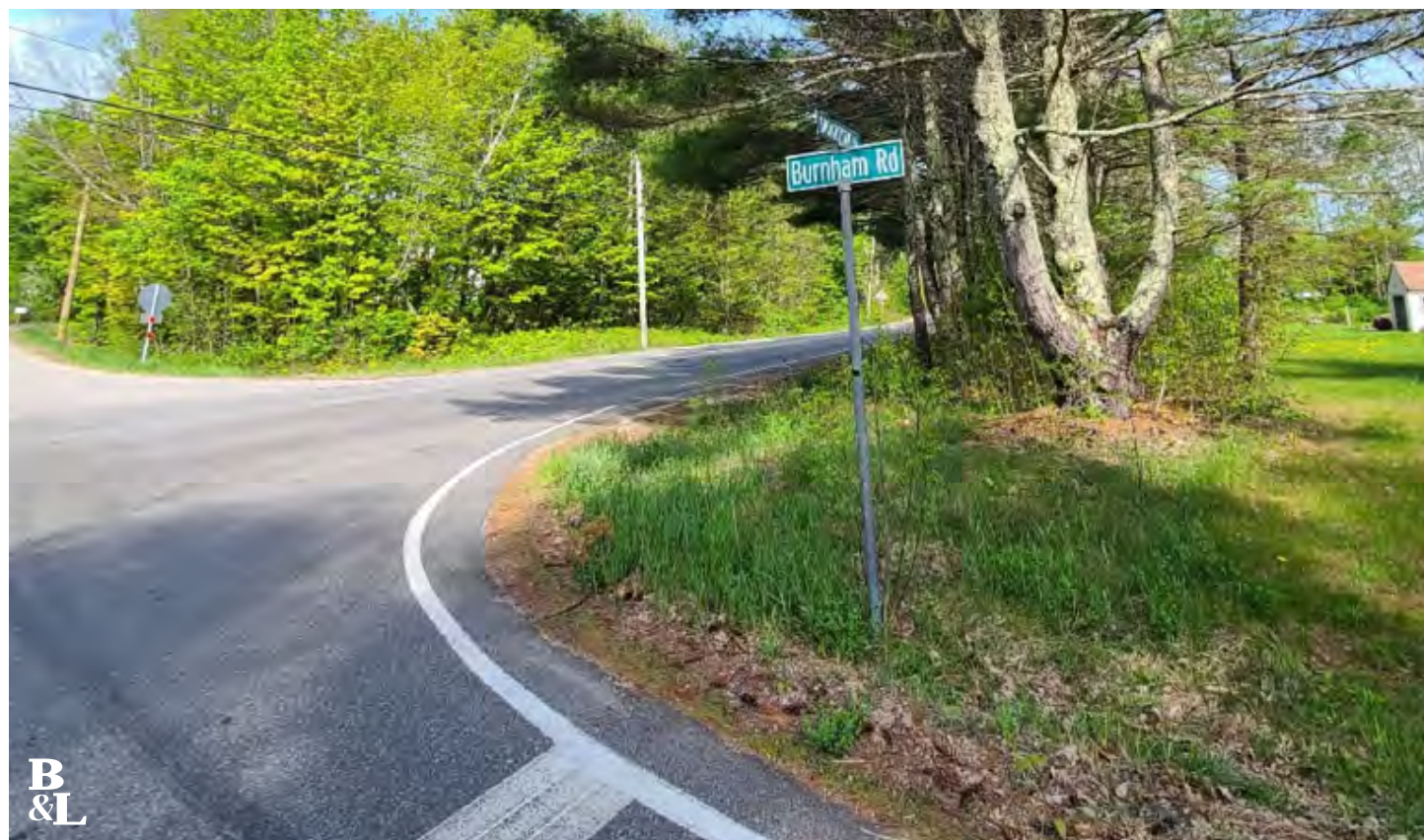
Figure 22 - Sight Distance Issue for Traffic Traveling Westbound on Burnham Road
