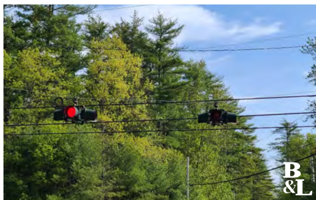
Figure 24 - Existing Flashing Beacon at Intersection of Broadturn Road and Holmes Road
