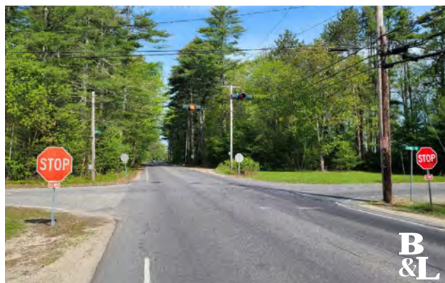
Figure 23 - Intersection of Broadturn Road at Holmes Road, Street View Facing North
