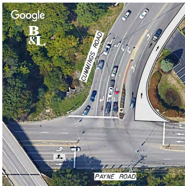
Figure 17 - Intersection of Payne Road at Cummings Road, Aerial View of Proposed Roadway Widening on Cummings Road to Accept Two Left-Turning Lanes
