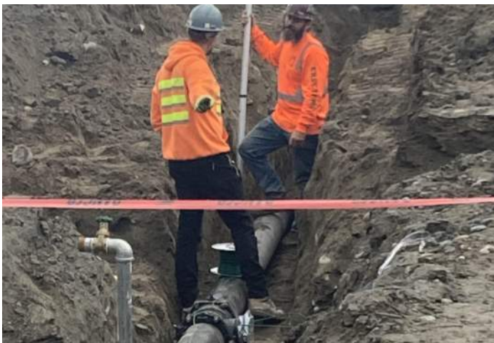
Water Main Installation
