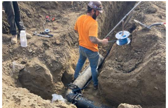
Water Main Installation
