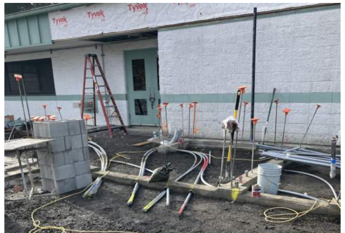
Under Slab Electrical Rough-In
