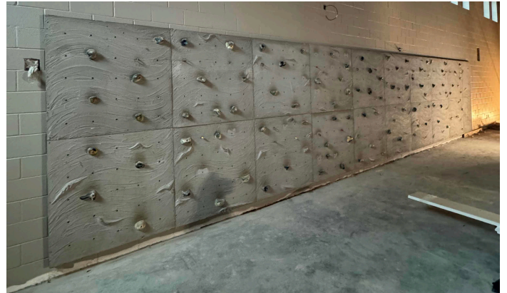
Rock climbing wall installed
