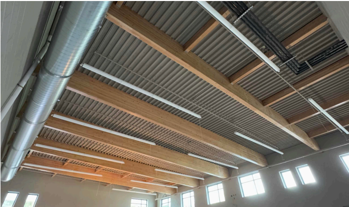
Gym light fixtures installed and beams sealed
