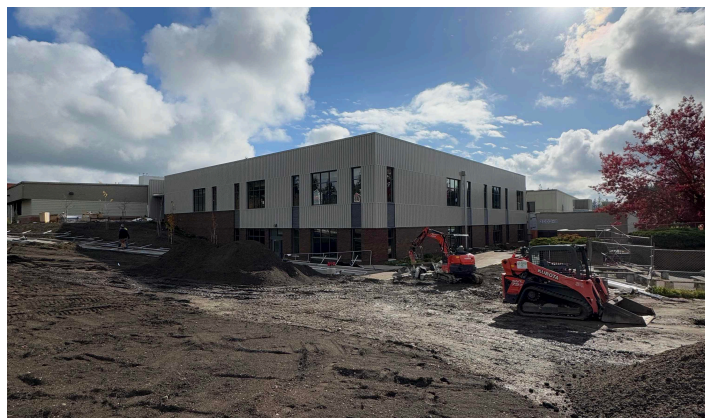
October construction progress
