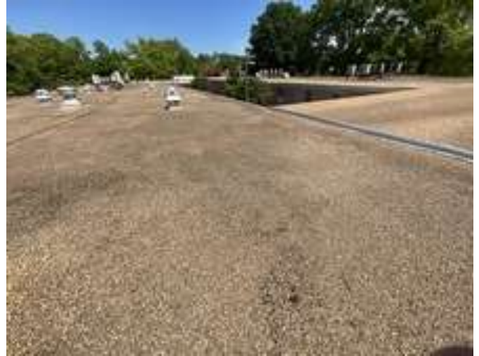
6 - PRIMARY ROOF OVERVIEW
