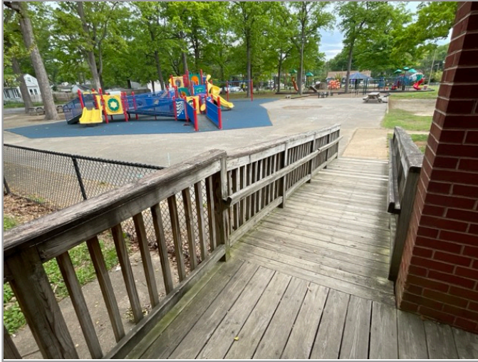
ACCESSIBLE ROUTE TO PLAYGROUND
