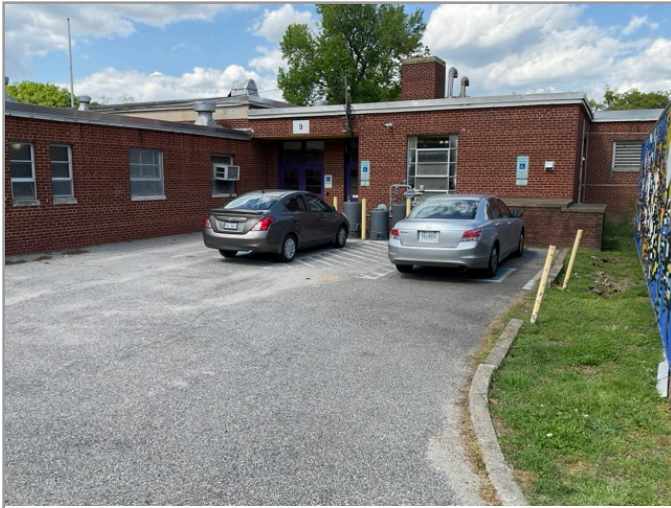
OVERVIEW OF ACCESSIBLE PARKING AREA
