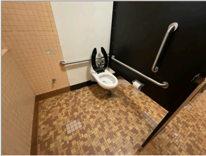
TOILET STALL OVERVIEW
