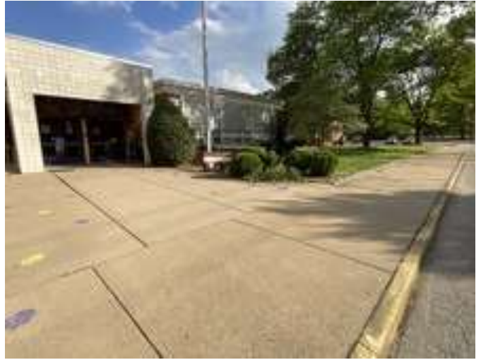
2 - SIDEWALKS AND LANDSCAPING
