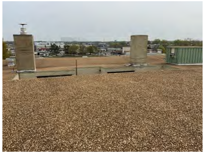
8 - SECONDARY ROOF OVERVIEW
