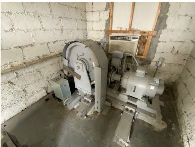
11 - OVERHEAD TRACTION ELEVATOR
