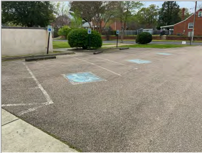
OVERVIEW OF ACCESSIBLE PARKING AREA
