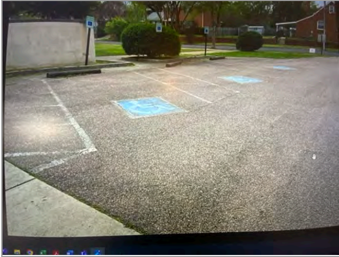
ACCESSIBLE ROUTE TO PLAYGROUND
