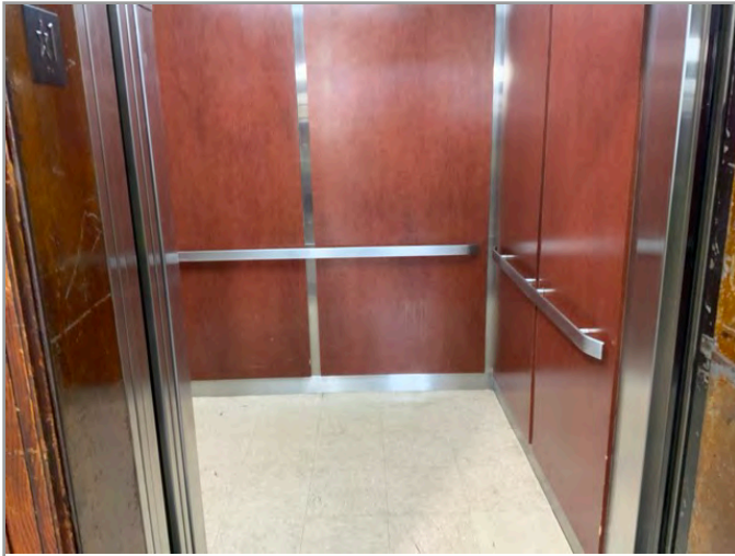
LOBBY LOOKING AT CABS (WITH DOORS OPEN)
