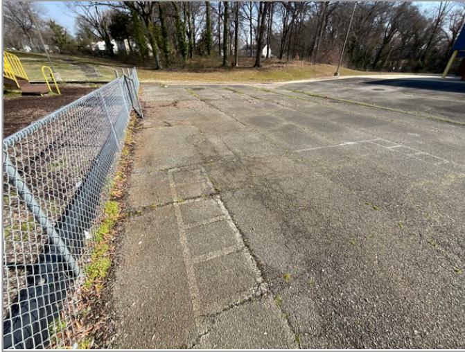
ACCESSIBLE ROUTE TO PLAYGROUND
