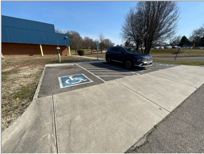
OVERVIEW OF ACCESSIBLE PARKING AREA
