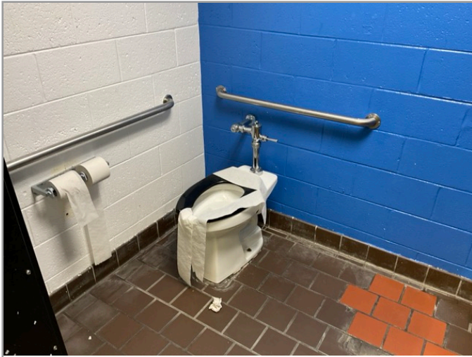
TOILET STALL OVERVIEW
