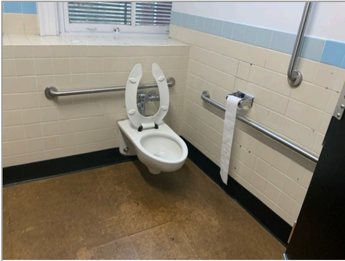
TOILET STALL OVERVIEW
