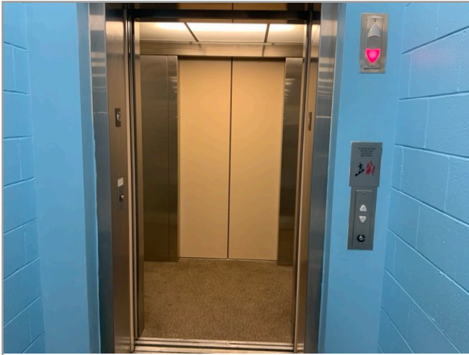
LOBBY LOOKING AT CABS
