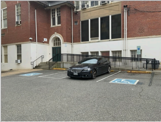
OVERVIEW OF ACCESSIBLE PARKING AREA
