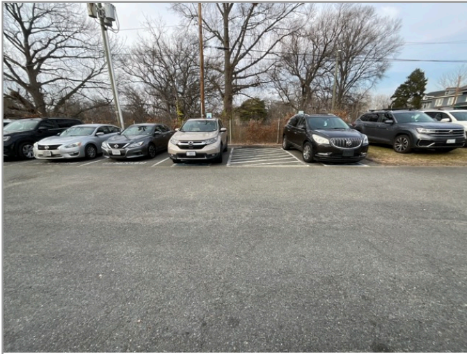
OVERVIEW OF ACCESSIBLE PARKING AREA
