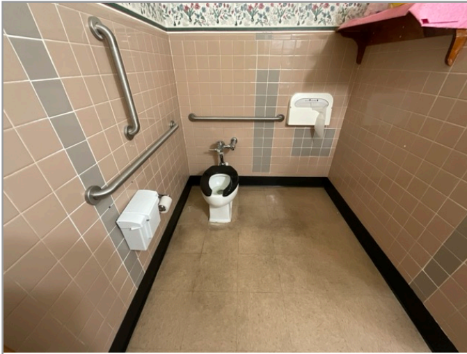
TOILET STALL OVERVIEW
