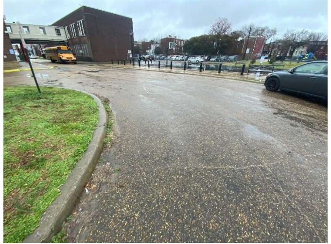
2 - DRIVE AISLE AND ADJACENT GROUNDS
