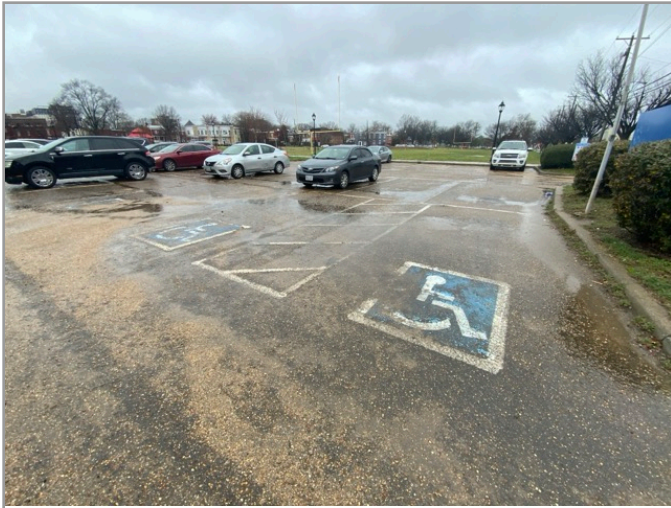
OVERVIEW OF ACCESSIBLE PARKING AREA
