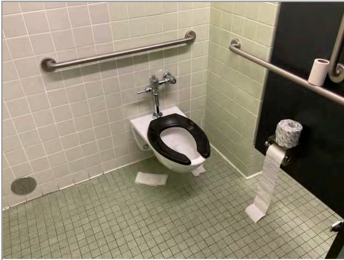
TOILET STALL OVERVIEW
