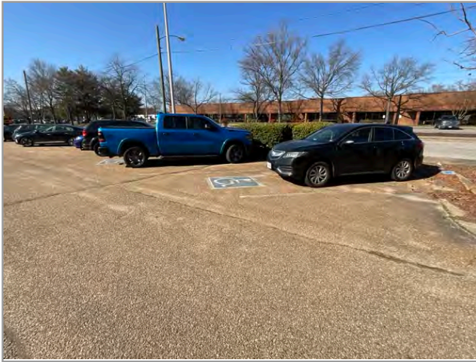
OVERVIEW OF ACCESSIBLE PARKING AREA
