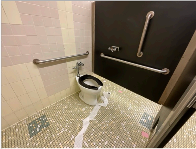
TOILET STALL OVERVIEW
