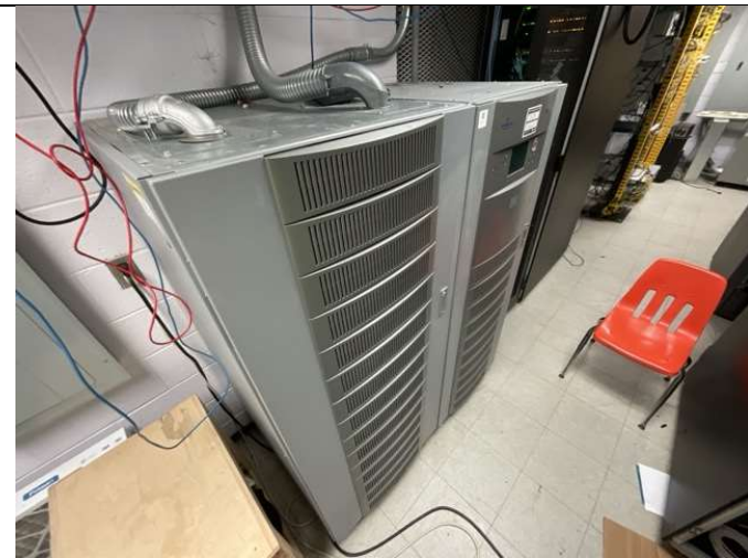
21 – UNINTERRUPTIBLE POWER SUPPLY
