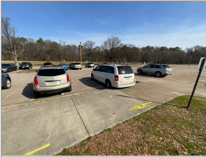
OVERVIEW OF ACCESSIBLE PARKING AREA
