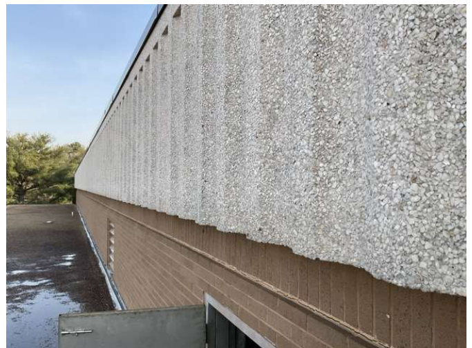
6 - BRICK AND CEMENT PANEL SIDING
