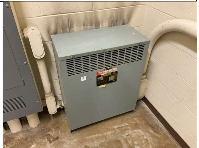
22 – SECONDARY TRANSFORMER
