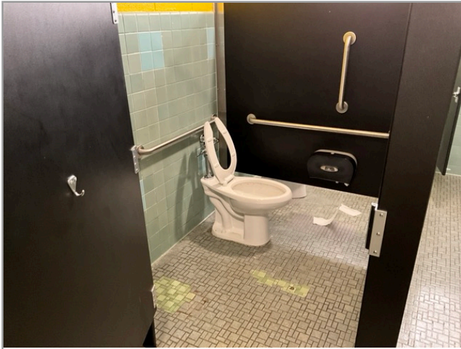
TOILET STALL OVERVIEW
