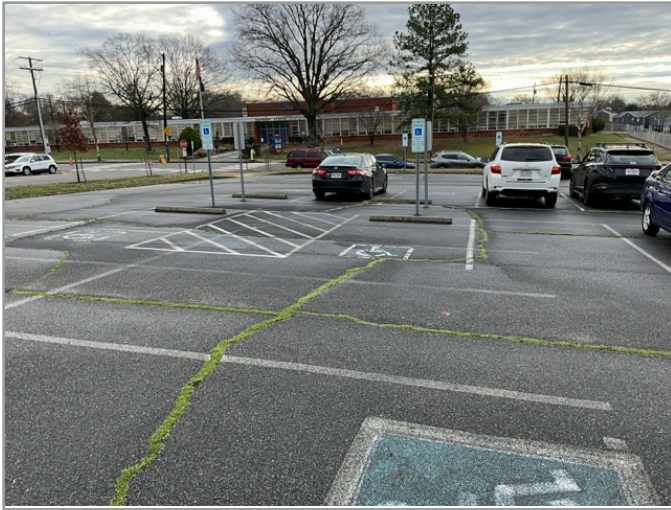
OVERVIEW OF ACCESSIBLE PARKING AREA
