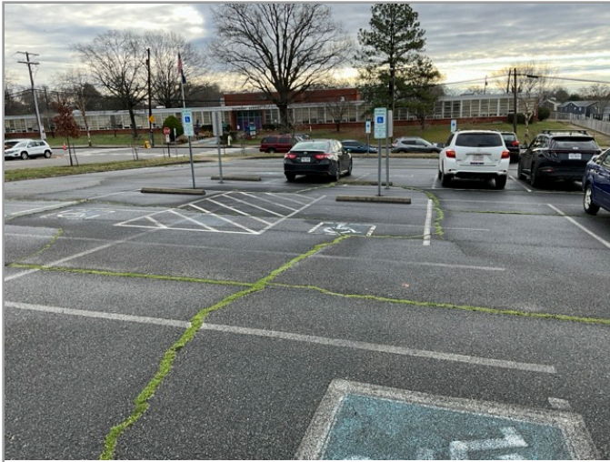
OVERVIEW OF ACCESSIBLE PARKING AREA
