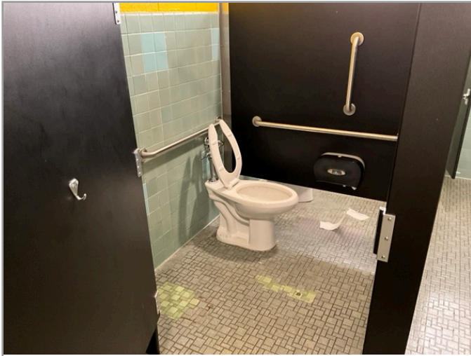
TOILET STALL OVERVIEW
