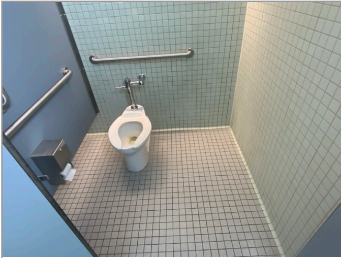
TOILET STALL OVERVIEW
