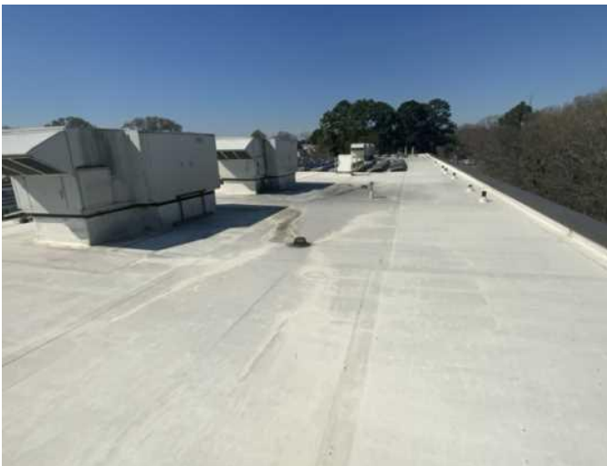
9 - PVC/TPO MEMBRANE ROOF
