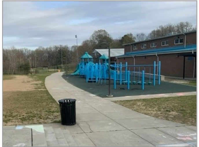
ACCESSIBLE ROUTE TO PLAYGROUND
