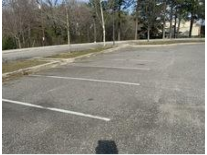
2 - ASPHALT PARKING LOT
