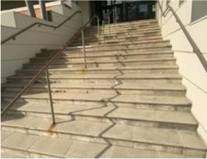
1 - PRECAST CONCRETE STAIRS
