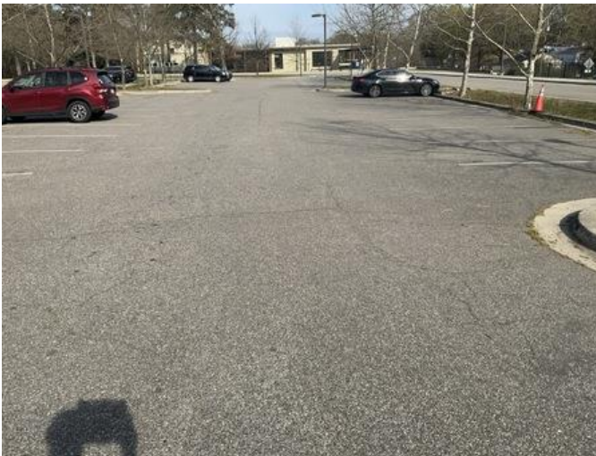
3 - ASPHALT PARKING LOTS
