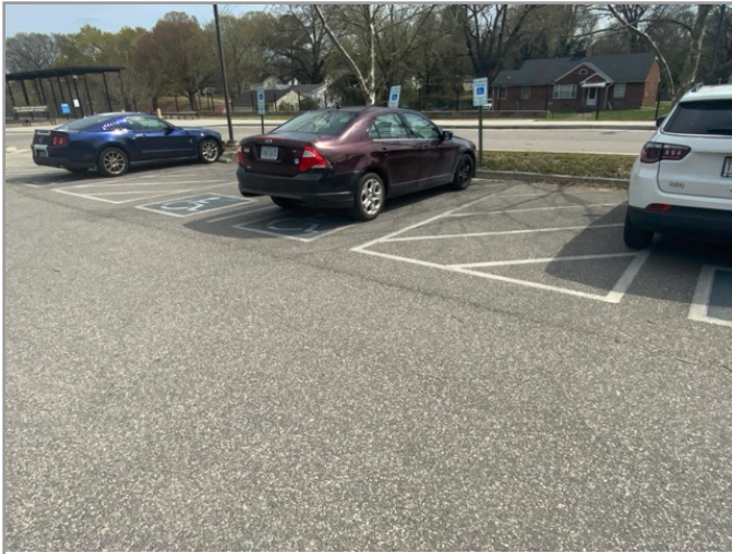
OVERVIEW OF ACCESSIBLE PARKING AREA
