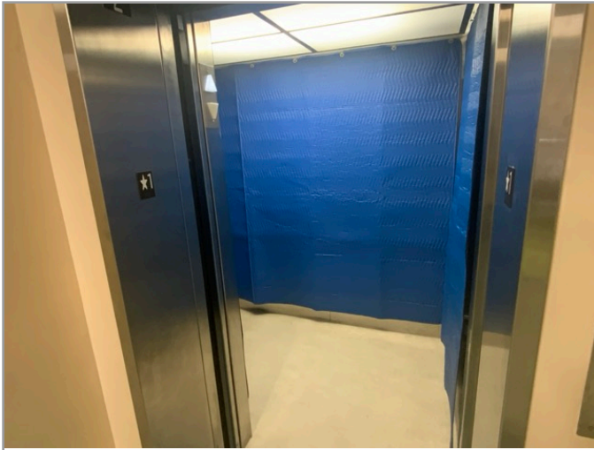
LOBBY LOOKING AT CABS
