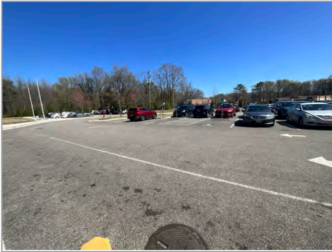
OVERVIEW OF ACCESSIBLE PARKING AREA
