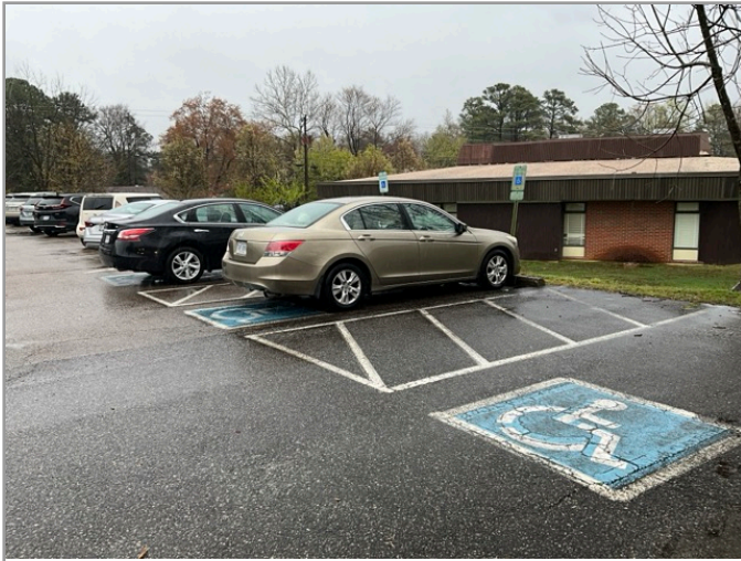
OVERVIEW OF ACCESSIBLE PARKING AREA
