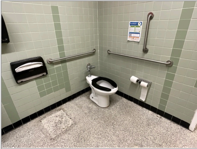
TOILET STALL OVERVIEW
