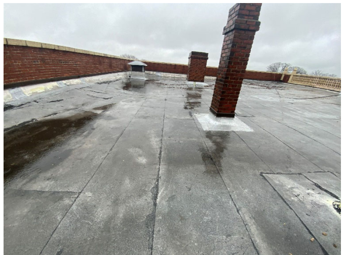
6 - MODIFIED BITUMEN ROOF
