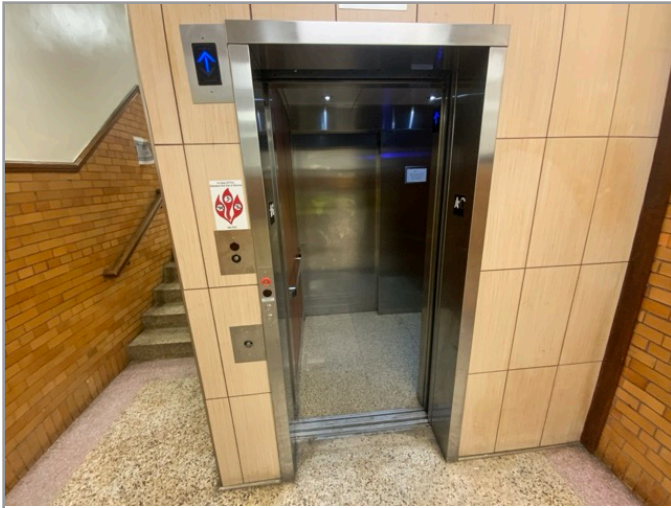
LOBBY LOOKING AT CABS
