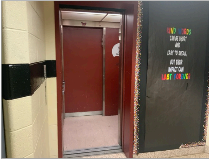
LOBBY LOOKING AT CABS
