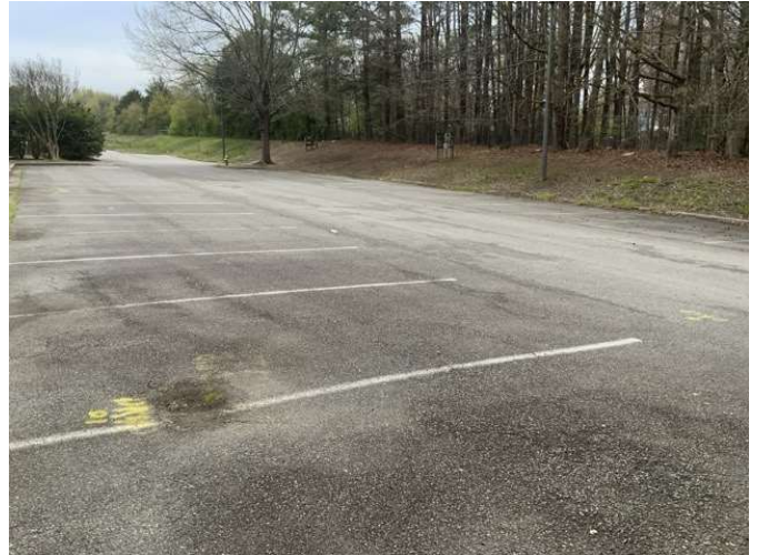
2 – REAR PARKING LOT
