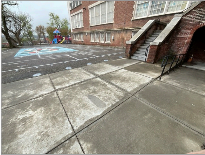
ACCESSIBLE ROUTE TO PLAYGROUND
