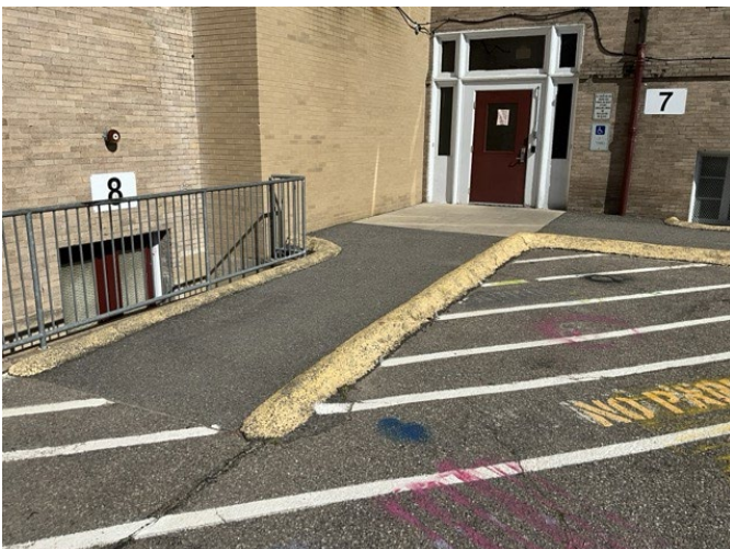
5 – PAINT AND STRIPING
