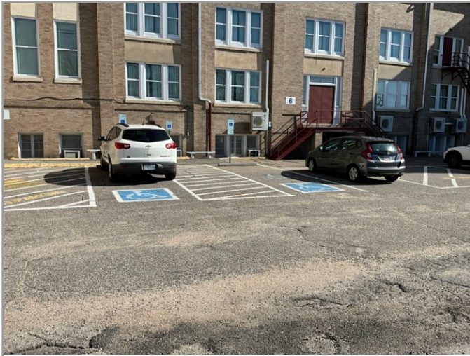
OVERVIEW OF ACCESSIBLE PARKING AREA
