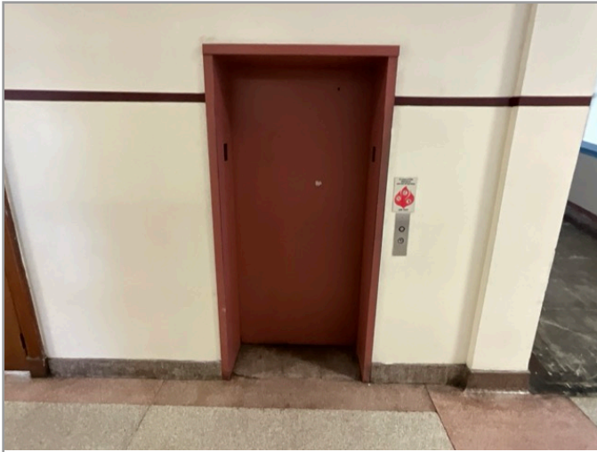
LOBBY LOOKING AT CABS
