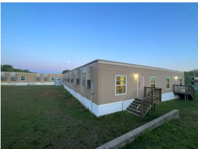
5 - SITE MODULAR BUILDING
