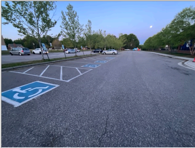
OVERVIEW OF ACCESSIBLE PARKING AREA
