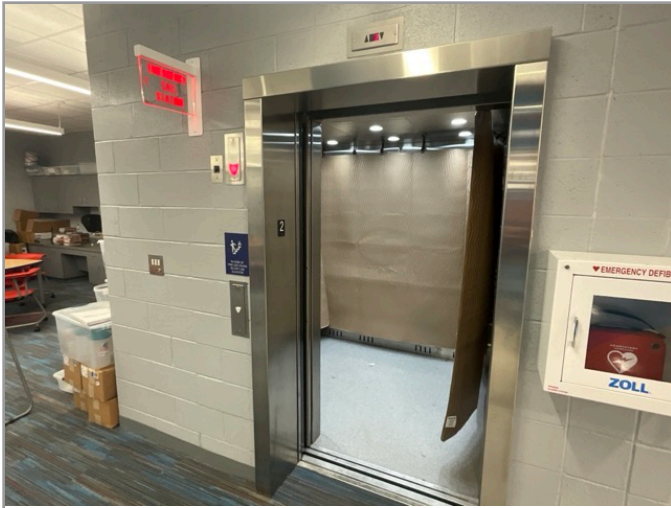
LOBBY LOOKING AT CAB
