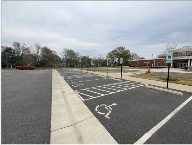
OVERVIEW OF ACCESSIBLE PARKING AREA
