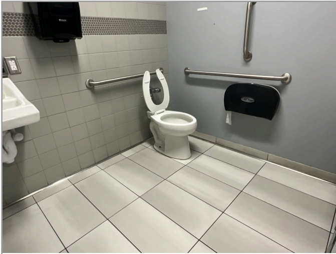
TOILET STALL OVERVIEW
