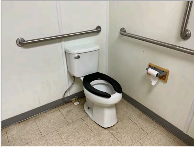
TOILET STALL OVERVIEW
