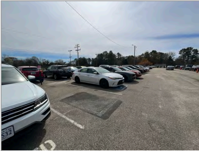
OVERVIEW OF ACCESSIBLE PARKING AREA
