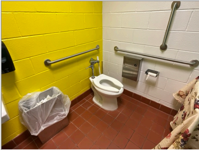
TOILET STALL OVERVIEW
