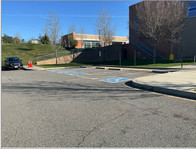
OVERVIEW OF ACCESSIBLE PARKING AREA
