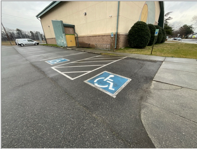
OVERVIEW OF ACCESSIBLE PARKING AREA
