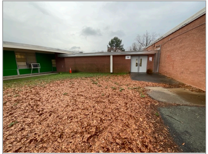
ACCESSIBLE ROUTE TO PLAYGROUND
