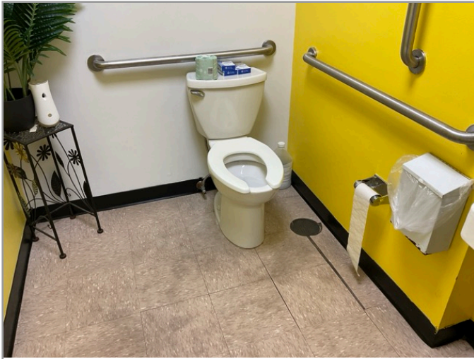
TOILET STALL OVERVIEW
