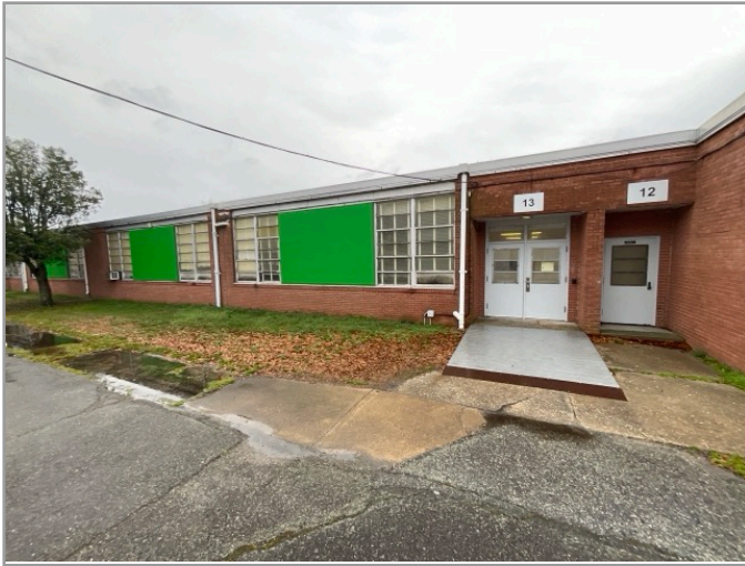
ACCESSIBLE ROUTE TO PLAYGROUND
