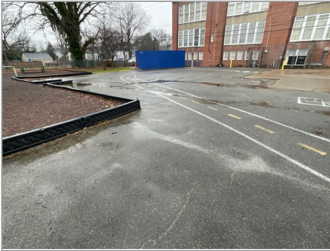
ACCESSIBLE ROUTE TO PLAYGROUND
