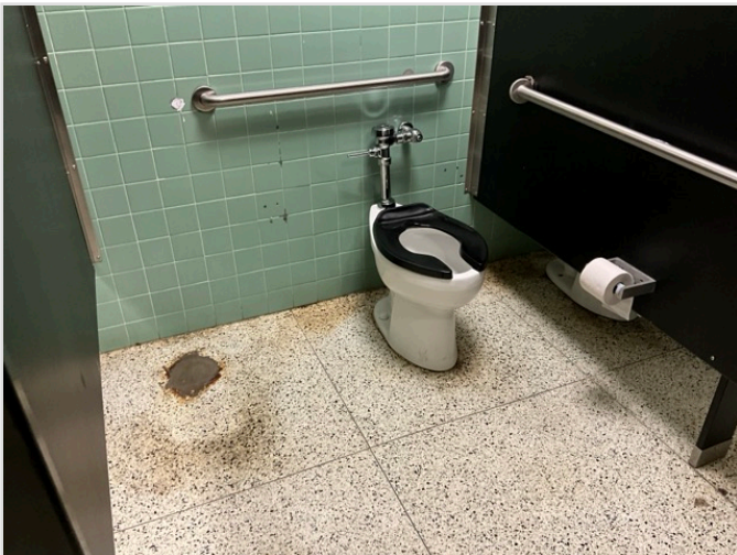
TOILET STALL OVERVIEW
