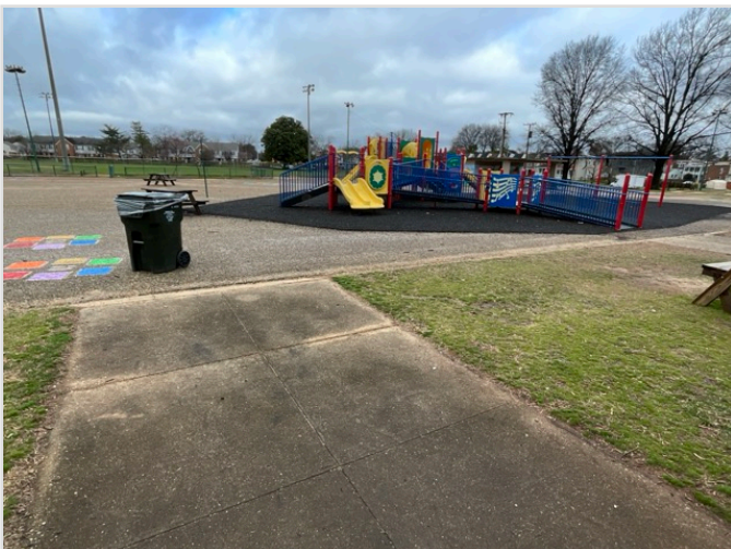
ACCESSIBLE ROUTE TO PLAYGROUND
